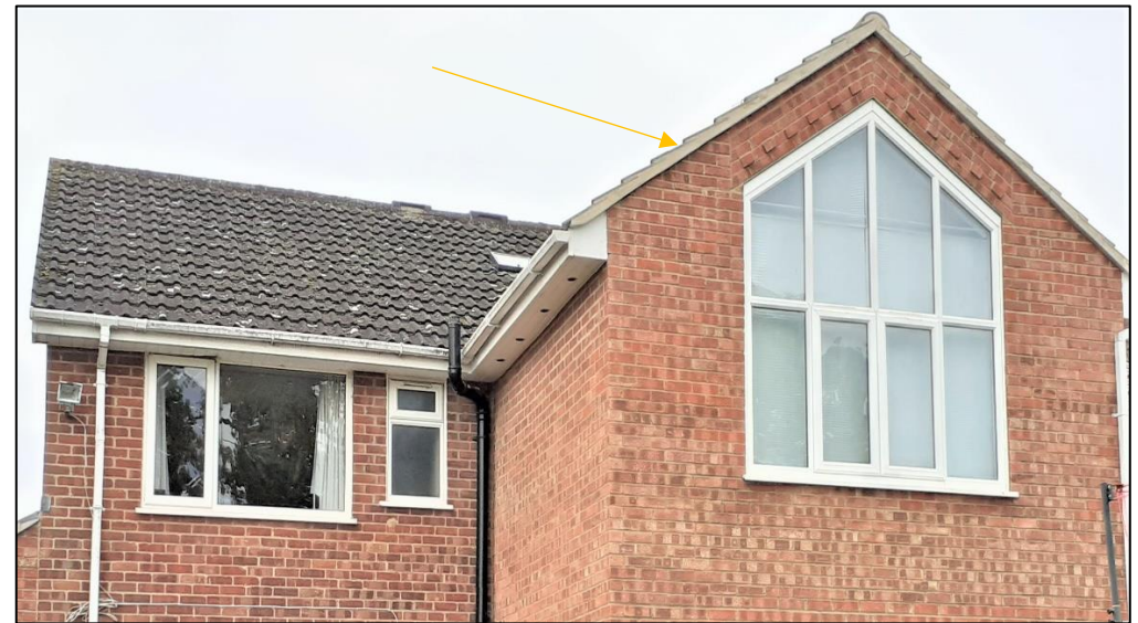
Photo 4: north-western elevation of B1.
