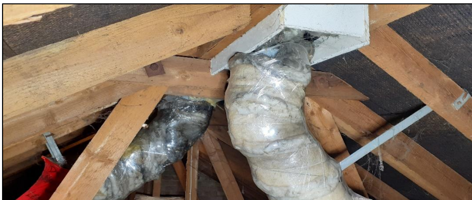
Photo 9: Internal – showing ducting which connects to the roof tile vents with no gaps.
