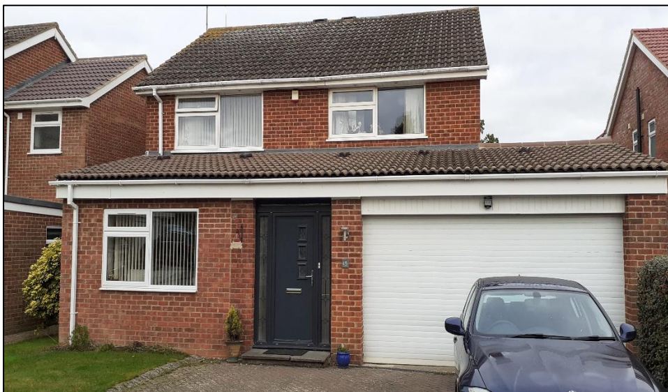
Photo 1: south-eastern elevation of B1.
