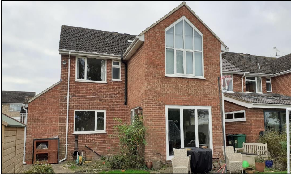
Photo 3: North-western elevation of B1.
