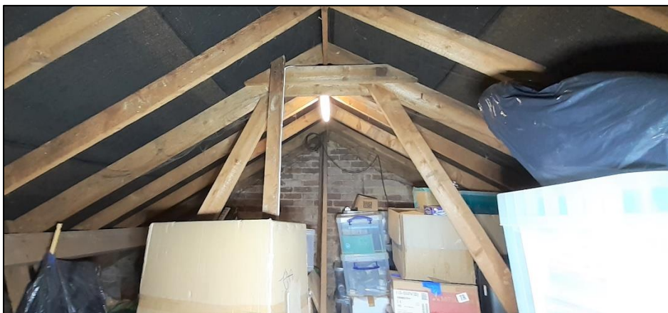
Photo 7: internal – looking west.
