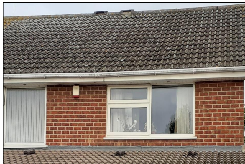
Photo 2: South-eastern elevation of B1.
