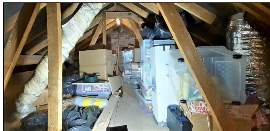
Photo 8: Internal – looking west.
