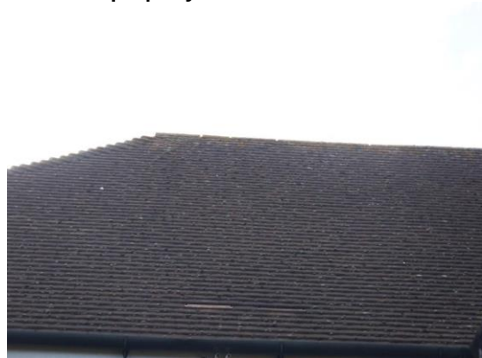
4. Flat overlapping roof tiles (rear elevation).
