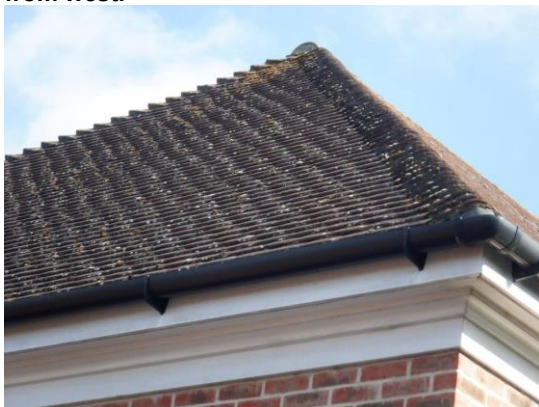
5. Mortared ridge and hip tiles (northern elevation).
