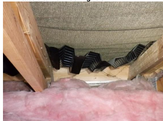
16. Open eave with visible soffit box.
