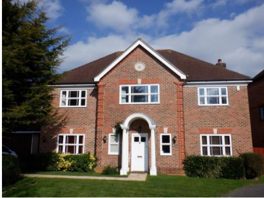
1. Front of property viewed from west.
