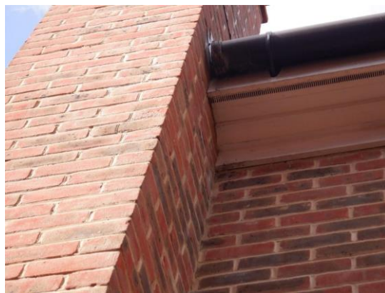
8. Soffit flush to chimney stack (southern elevation).
