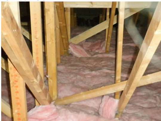
15. Fibreglass floor insulation.
