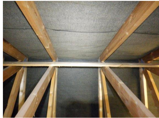
14. Intact bitumen roofing felt.
