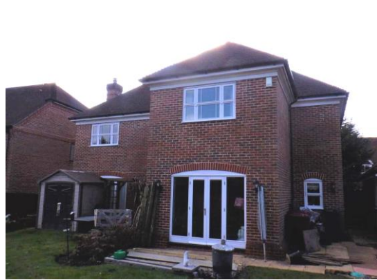
2. Rear of property viewed from east.
