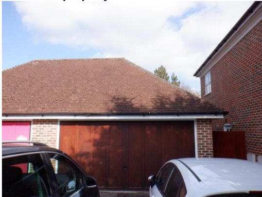
3. Front of shared detached garage viewed from west.
