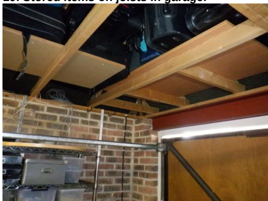
21. Tight timber wall plate on garage walls.
