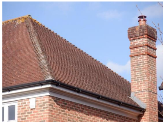
6. Mortared ridge and hip tiles (southern elevation).
