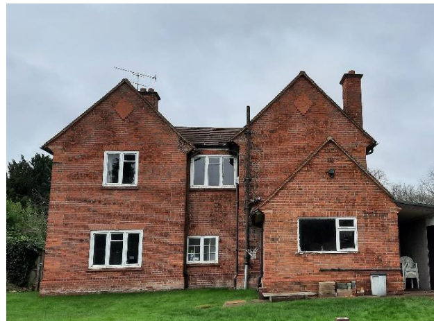
Plate 4.2: Rear of building (north-east elevation)
