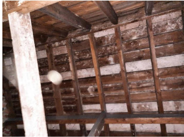
Plate 4.21: Loft void above kitchen extension
