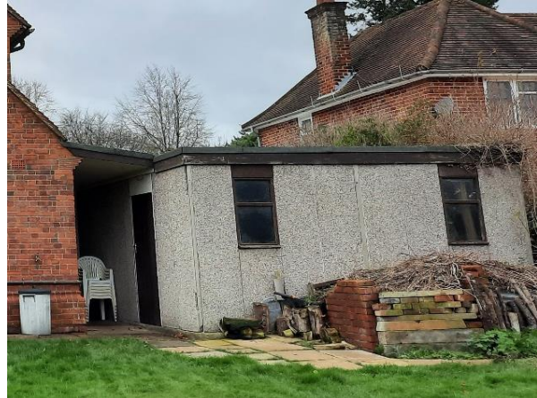
Plate 4.24: Rear of garage (north-east elevation)
