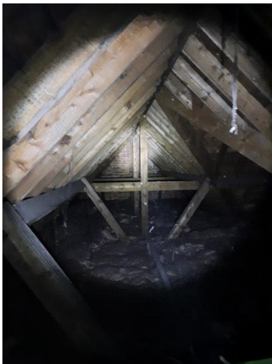
Plate 4.15: Main loft void with fibre glass insulation
