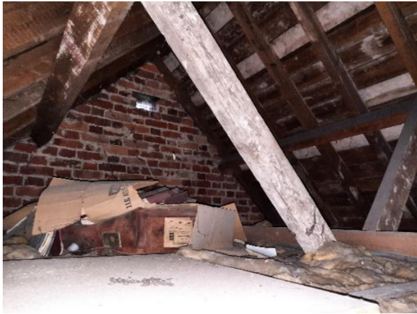
Plate 4.20: Loft void above kitchen extension
