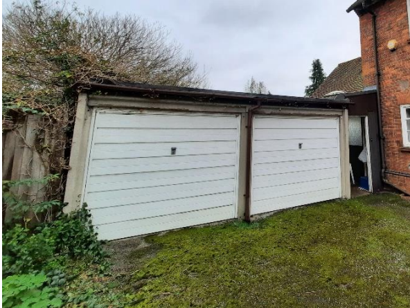
Plate 4.23: Front of garage (south-west elevation)
