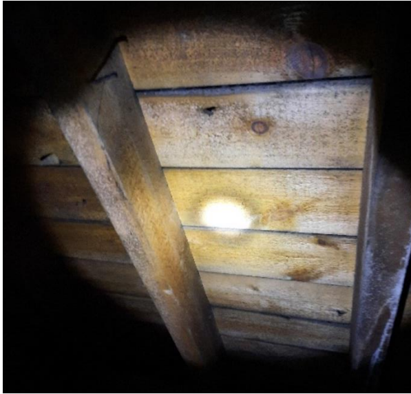
Plate 4.17: Wooden sarking boards on wooden ridge beams
