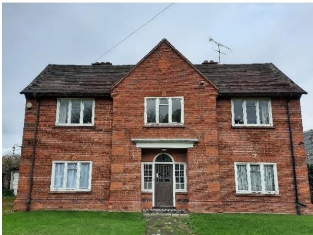
Plate 4.1: Front of building (south-west elevation)
