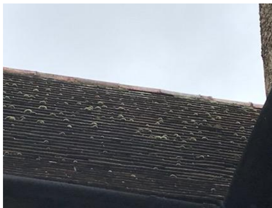
Photograph 6: Gaps under the ridge tiles on the southern elevation
