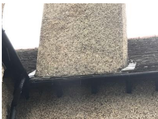
Photograph 5: Lifted tiles on the lean-to extension
