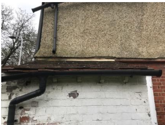
Photograph 5: Lifted tiles on the lean-to extension
