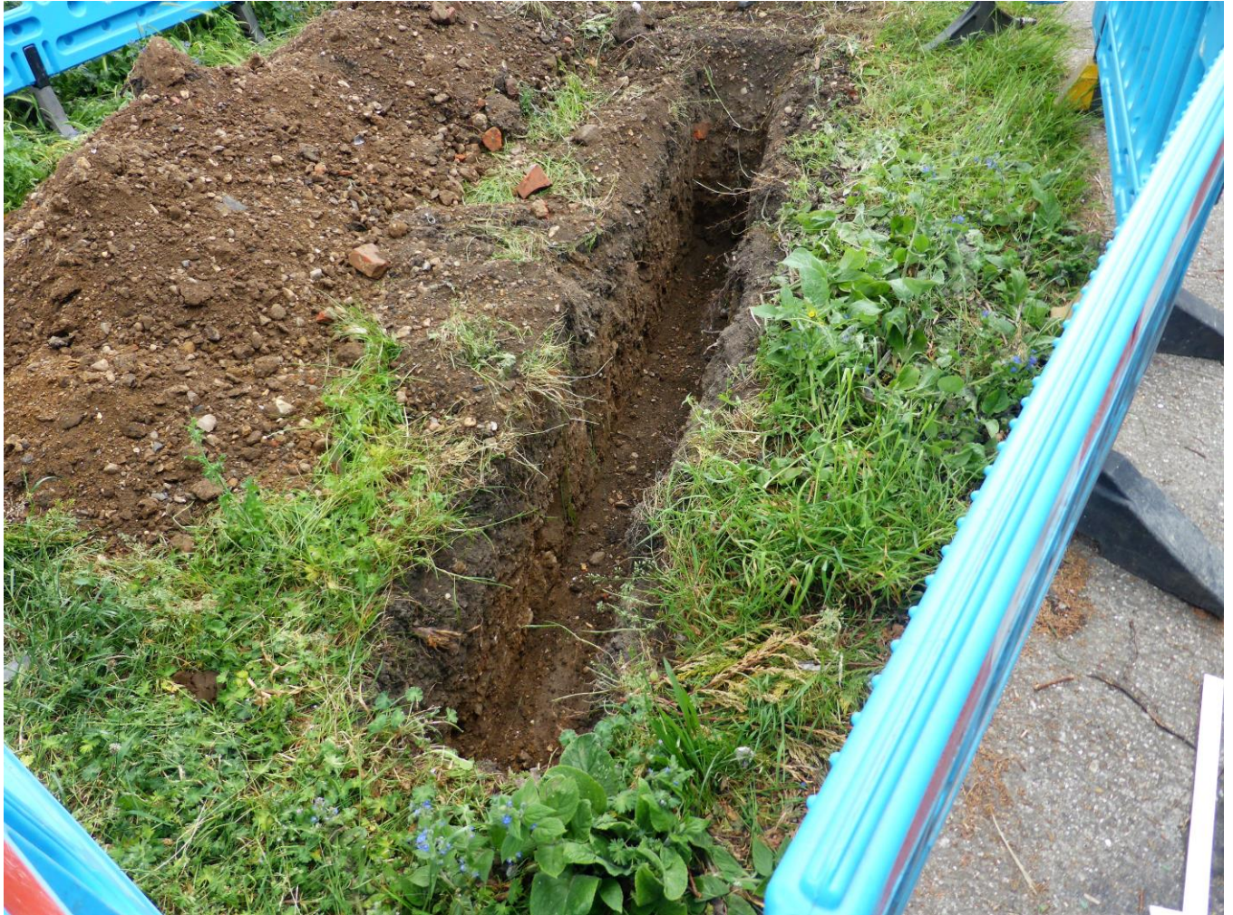
TRENCH 'A' - ERLEIGH ROAD FRONTAGE
