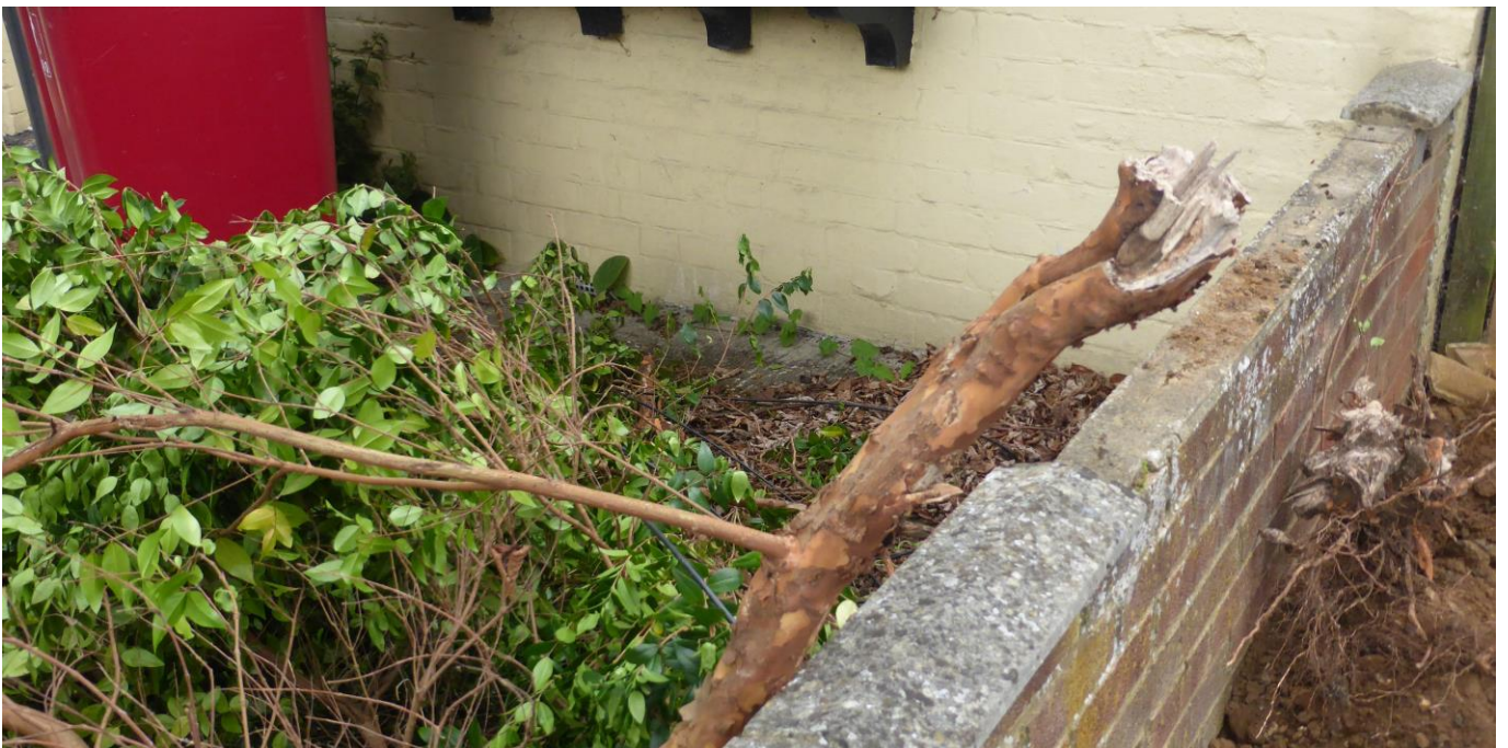
BUSH REMOVED TO ALLOW DIGGING OF TRENCH 'B'
