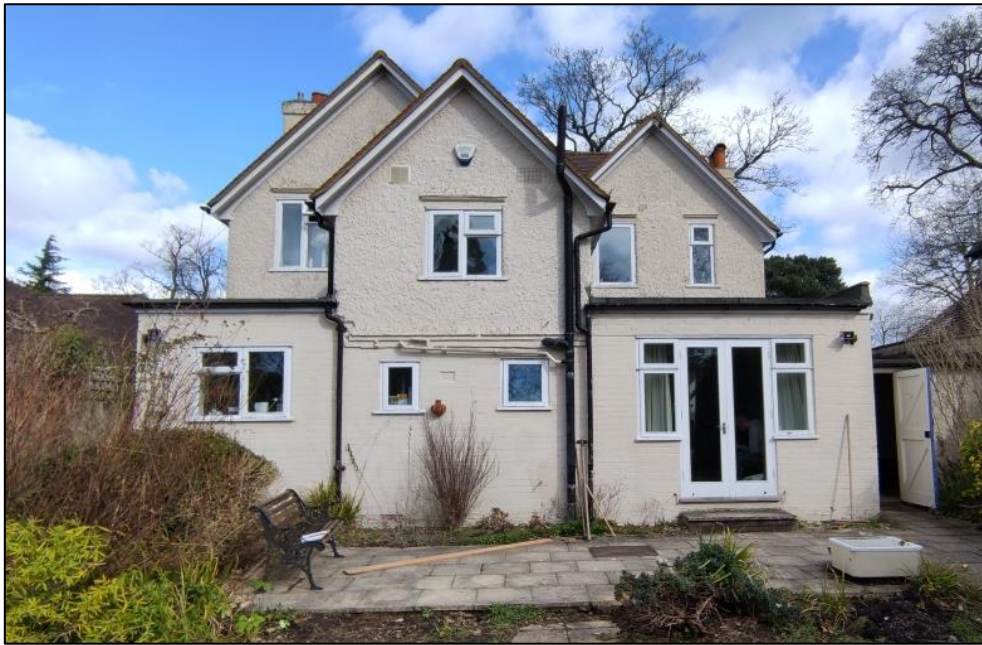
Figure 3 – Rear (western) elevation of 20 Shinfield Road
