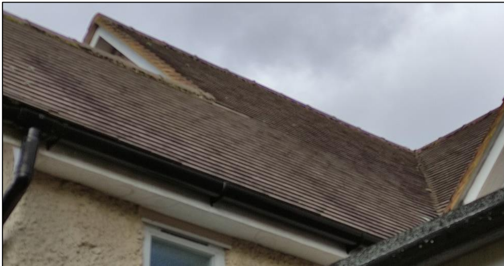
Figure 7 – roof showing tightly fitting machine-made clay tiles and sealed soffits
