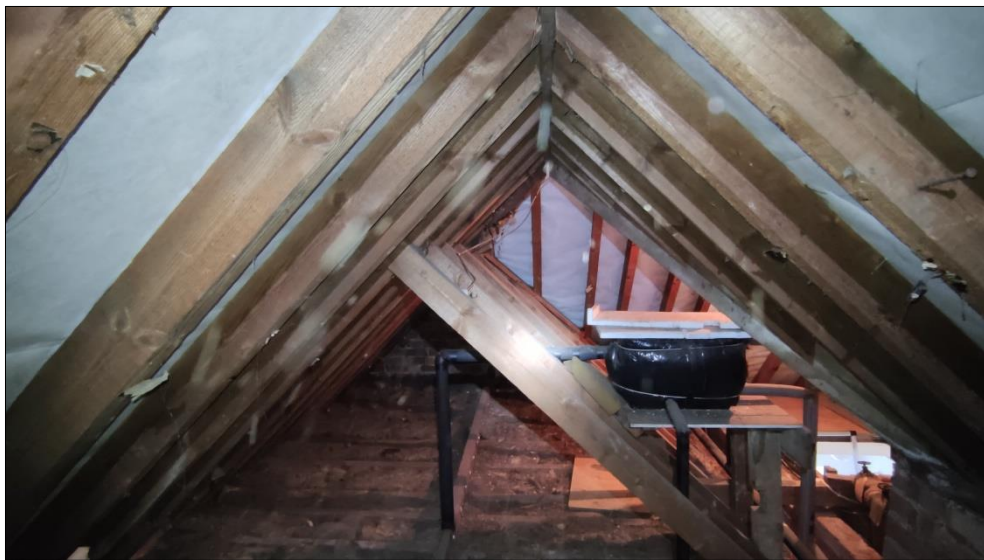
Figure 6 – showing the section of roof running along the northern elevation
