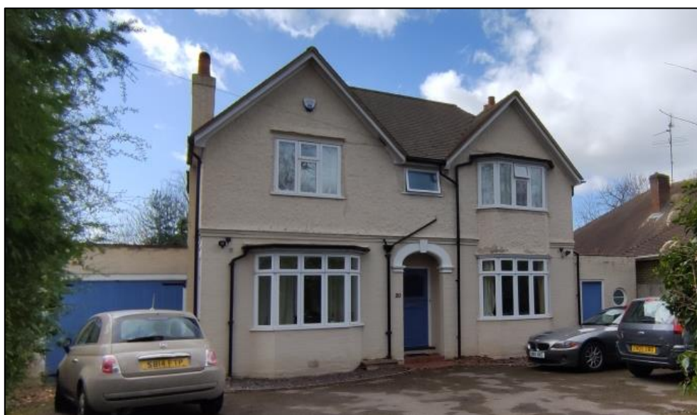
Figure 2 - Front (eastern) elevation of 20 Shinfield Road
