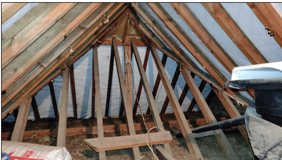
Figure 4 – showing central section of the roof void with access to other areas
