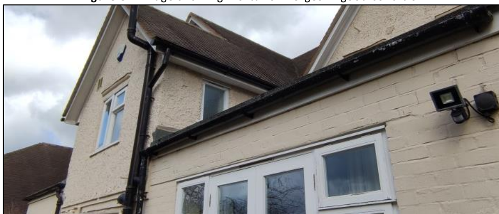
Figure 9 – showing flat roofs on extensions in good condition, with tightly fitting weatherboarding
