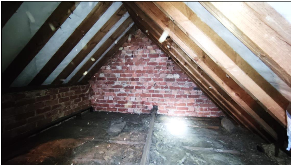
Figure 5 – showing excellent condition of breathable membrane and gable end brickwork
