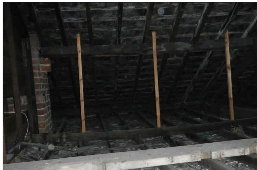
Photograph F : Loft space of building 87A/88
