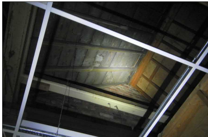
Photograph H : Internal view of multiple pitch roof at south of building 87A
