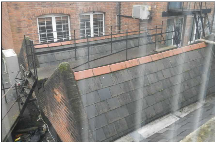
Photograph G : Single storey section at south of building 87A
