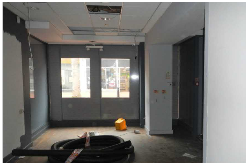
Photograph D : Ground floor of building B87A
