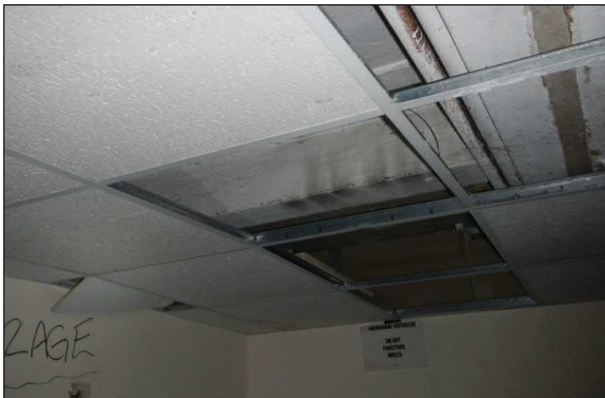
Photograph E : Basement of building 87A
