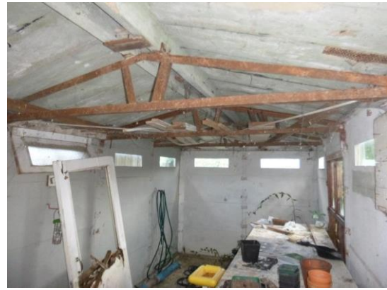
20. Pre-fab shed interior.
