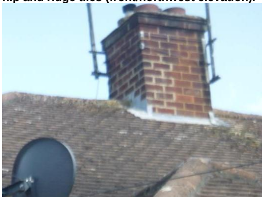
5. Tight lead flashing around chimney (front elevation).
