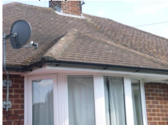
4. Tight hipped end above bay window (front elevation).
