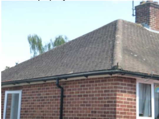
3. Flat overlapping roof tiles and fully mortared hip and ridge tiles (front/northwest elevation).
