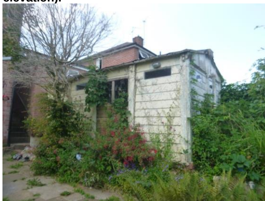
10. Neglected pre-fab shed (southeast elevation).
