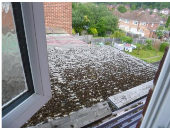
7. Corrugated asbestos cement roof on garage viewed from house window.
