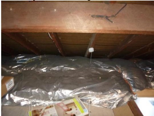
15. Foil-wrapped fibreglass floor insulation and exposed eaves.
