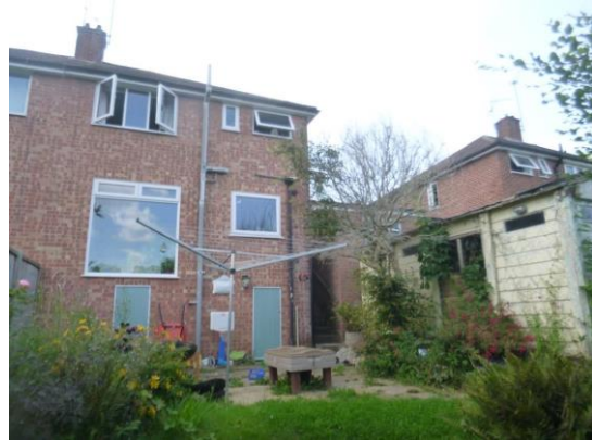
2. Rear of property viewed from east.
