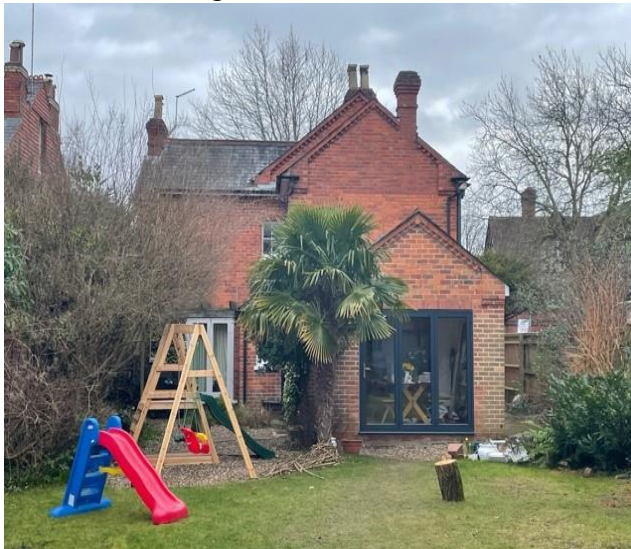
Photo 1. Existing rear elevation
