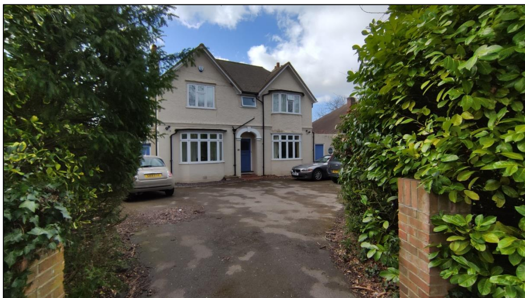
Figure 3 – view from site boundary showing bushes, tarmacked driveway/parking and detached house
