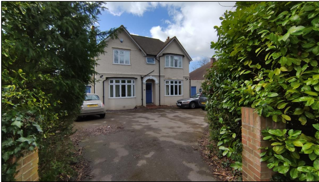
Figure 8a – Showing hard-standing area at the front of the property
