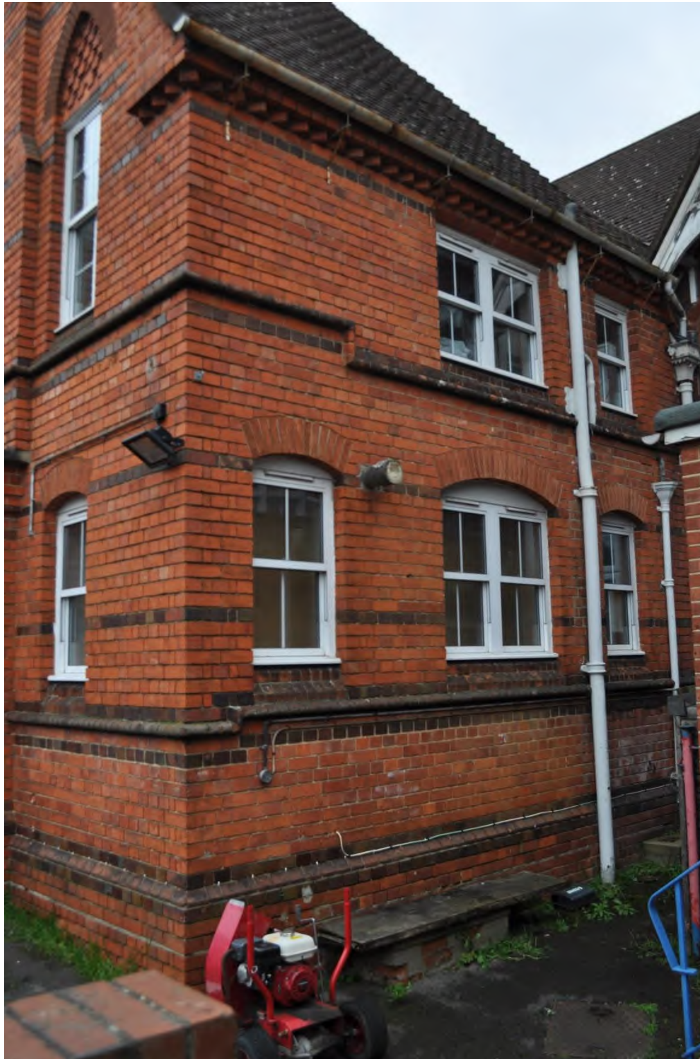
1.4.1, 1.4.2 South Elevation 2 Brickwork and 1.5.3 Downpipes
