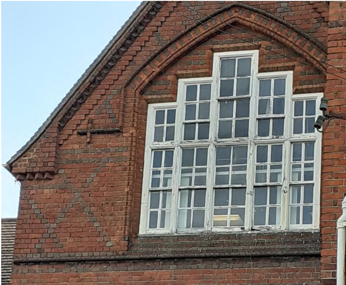
1.4.3 West Elevation 2 Brickwork W1 Gable
