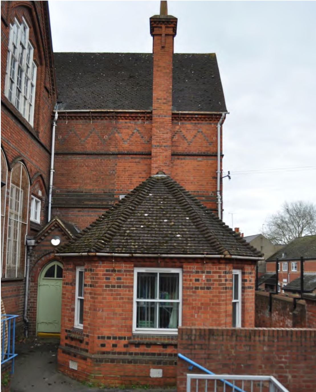
1.4.5 West Elevation 2 Brickwork chimney wall
