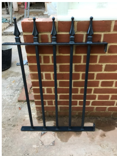
Fig 4: PPC Steel railings sample panel
