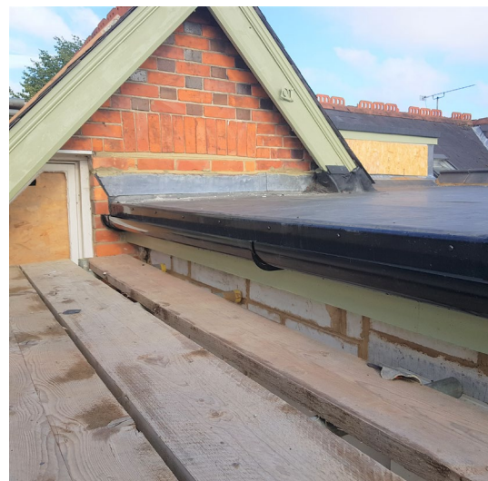
Fig 5: Half round black uPVC gutter to match existing
