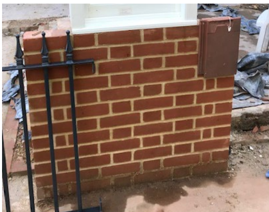
Fig 1: Imperial size Chelmer red brick sample panel Fig 2: Timber sash window frame, sill, surround & glazing sample
