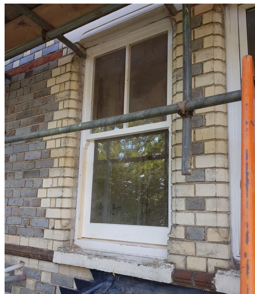
Fig 1: Imperial size Chelmer red brick sample panel Fig 2: Timber sash window frame, sill, surround & glazing sample
