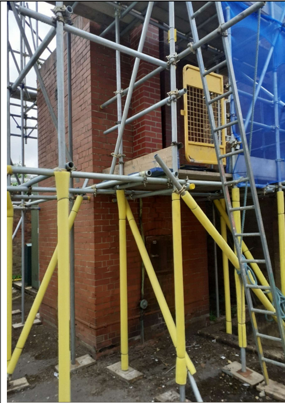
Figure 3. View from ground level. Lower rectangular part with access hatch.
