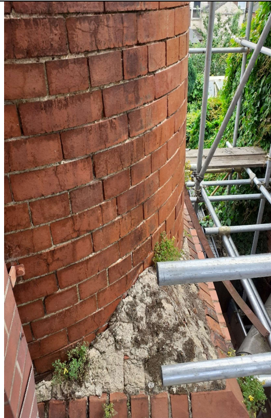
Figure 4. View from first level. Interface detail between upper circle and lower rectangle.
