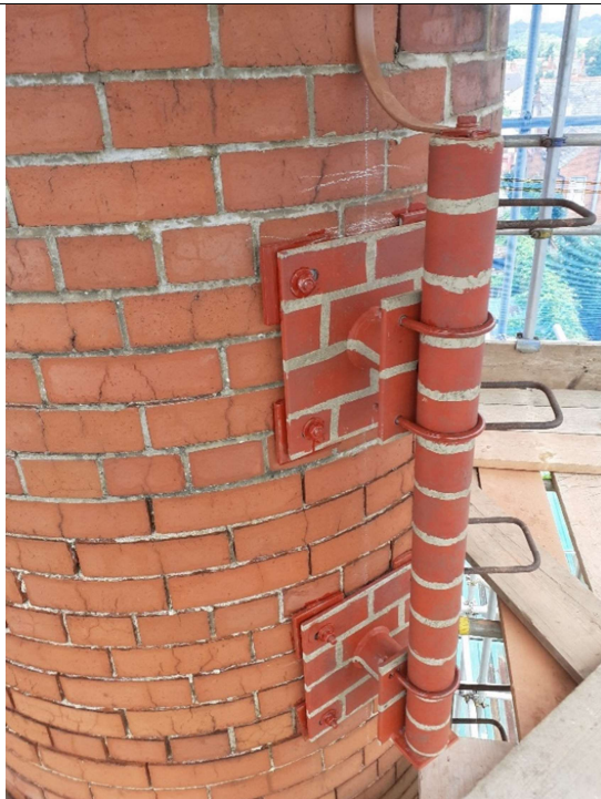
Figure 7. View from scaffolding level 4. Painted wall plates with resin anchors (front), existing U-bars acting as ladder steps (back)
