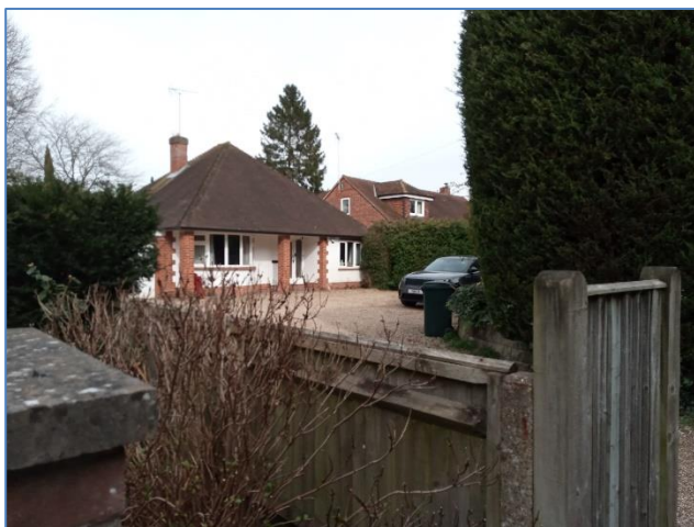
1. Front of 21 Derby Road. Photo taken on 08/03/2021.
