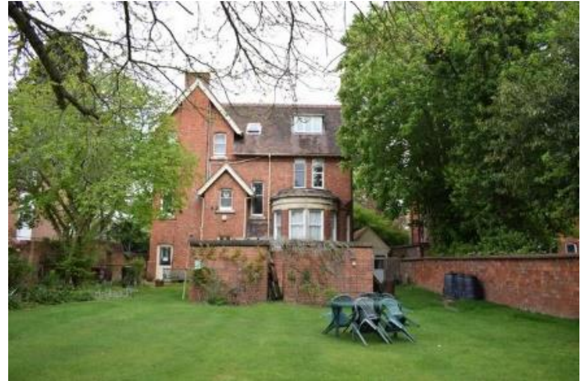
Plate 2: Looking north at the rear elevation of Number 9
