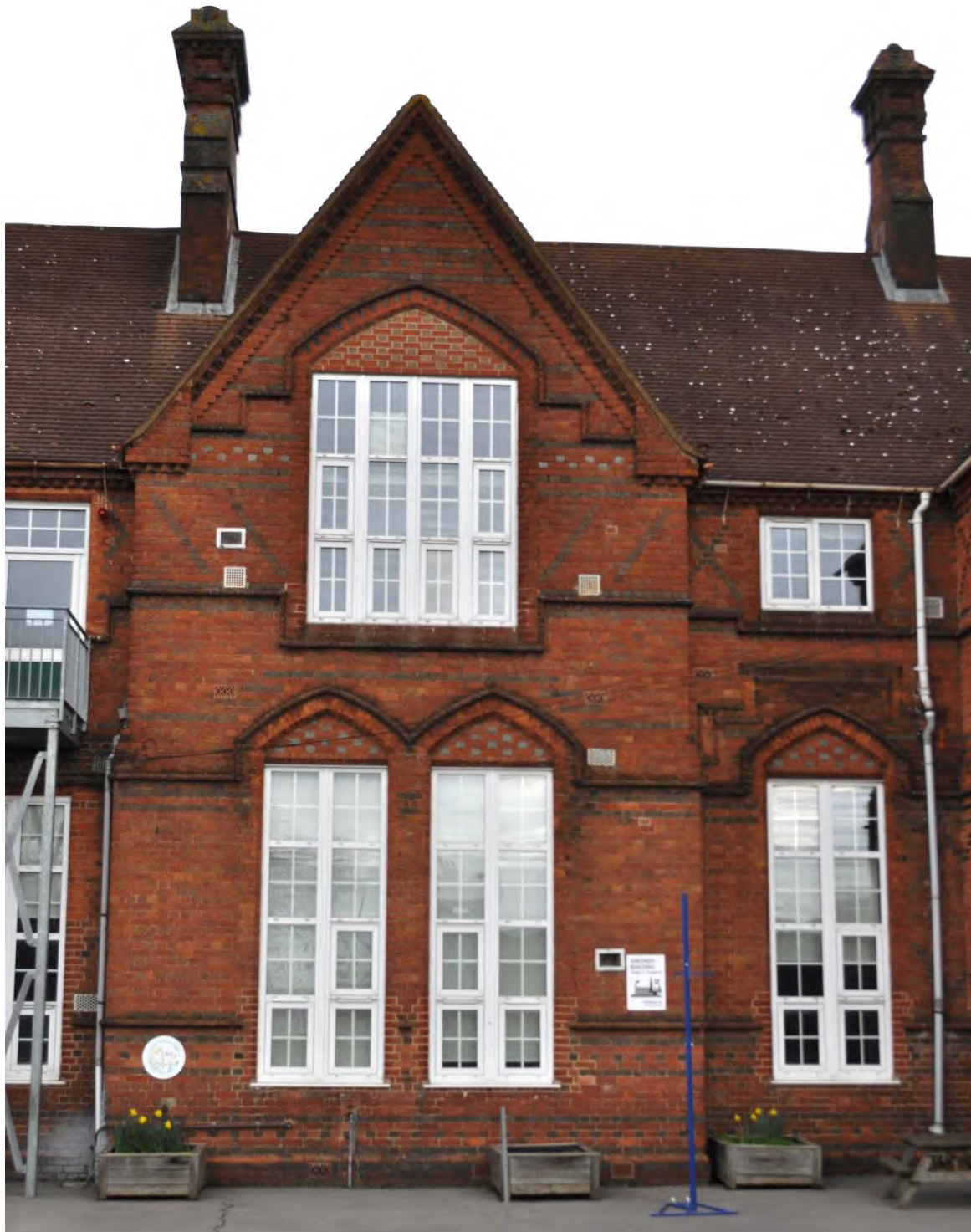
3.4.6 South Elevation 1 LH Gable Brickwork
