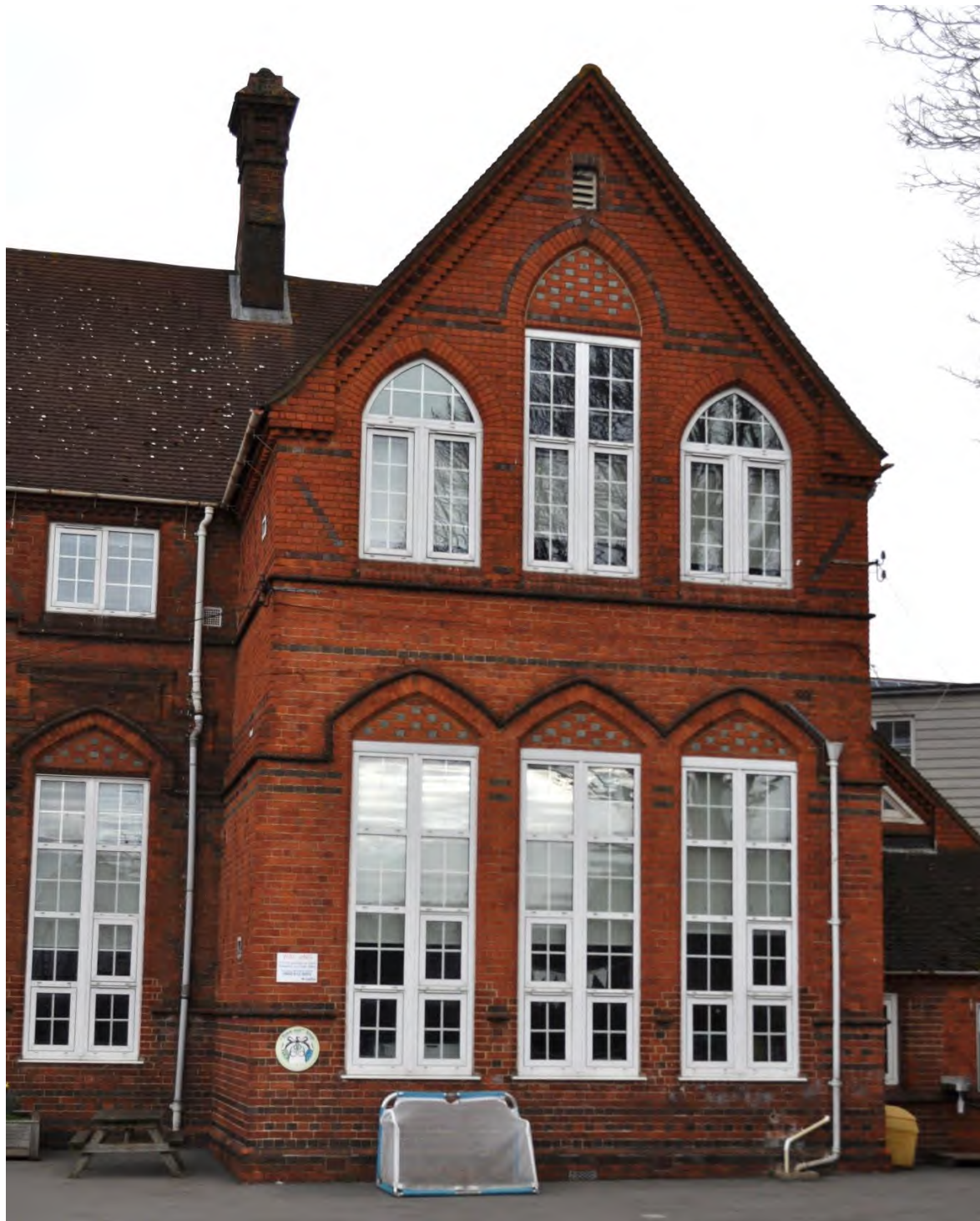
3.4.9 -.10 South Elevation 1 Between and RH Gable Brickwork
