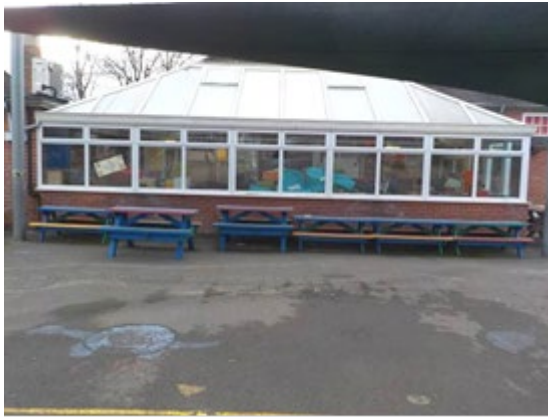
North Elevation of existing Conservatory
