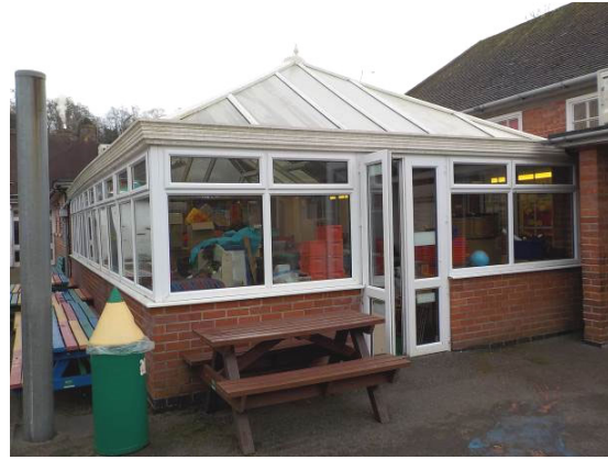
West Elevation of existing Conservatory
