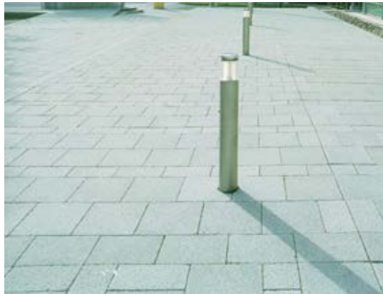
Concrete flag surfacing to demarcate building entrance.
