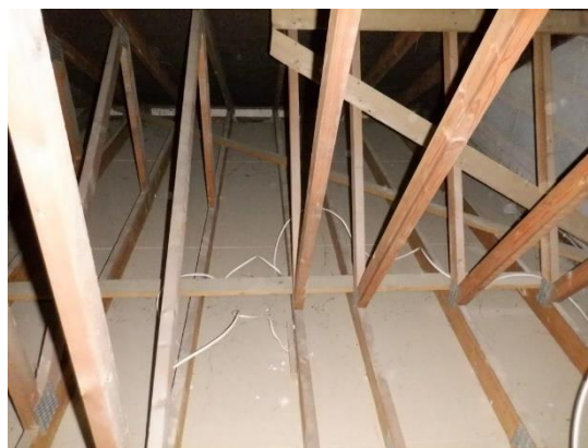
18. Second roof void above the garage.
