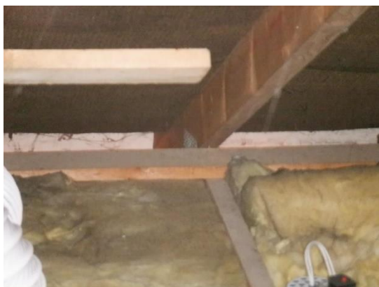
15. Eaves open into the soffits.
