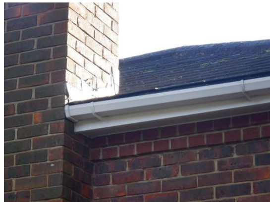
6. Tight lead flashing and sealed soffit to chimney stack (north elevation).
