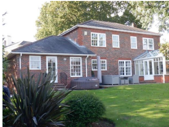
2. Rear of house viewed from the east.
