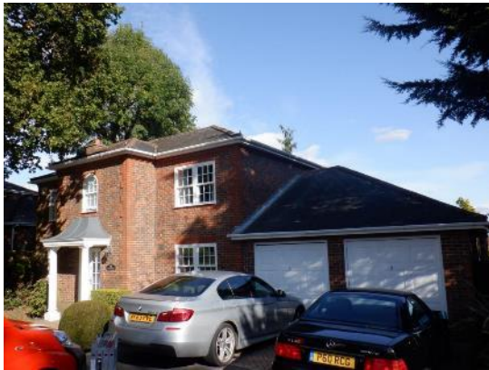
1. Front of house viewed from the west.
