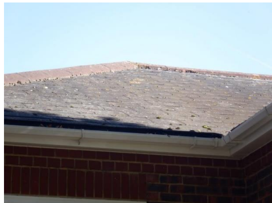
4. Tight ridge and hip tiles with intact mortar.
