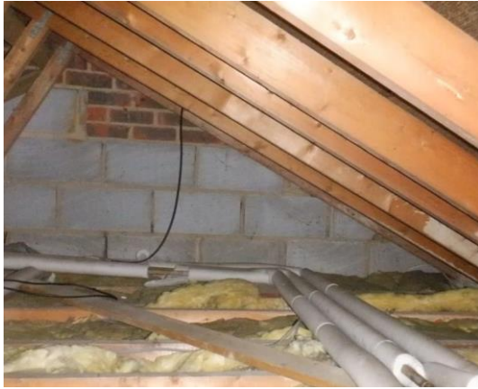
19. Part block and part brickwork wall of the house.
