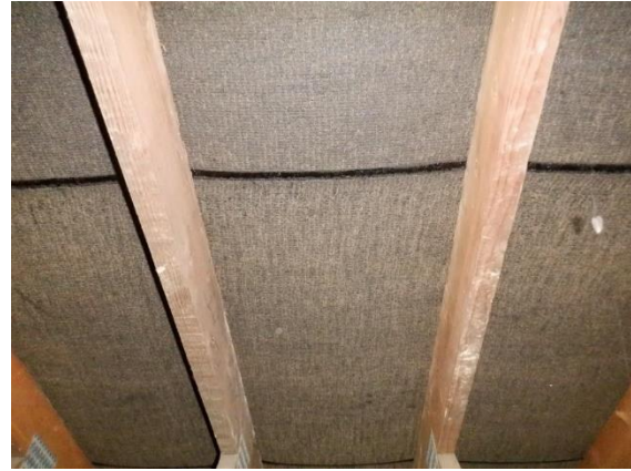
20. Roof lined with hessian and bitumen roofing felt.
