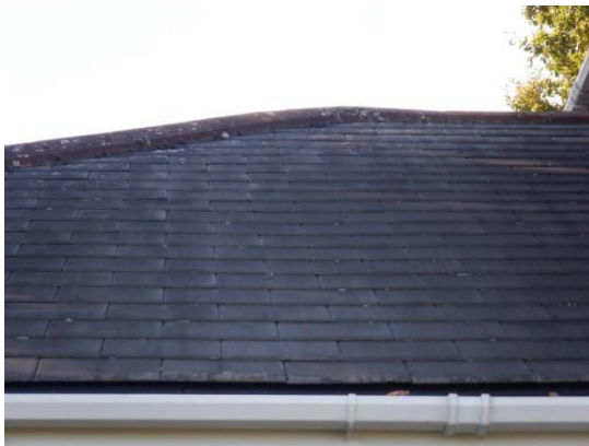
3. Flat slate roof tiles (rear elevation).
