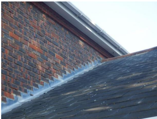
5. Tight lead flashing where the garage roof joins the house (front elevation).
