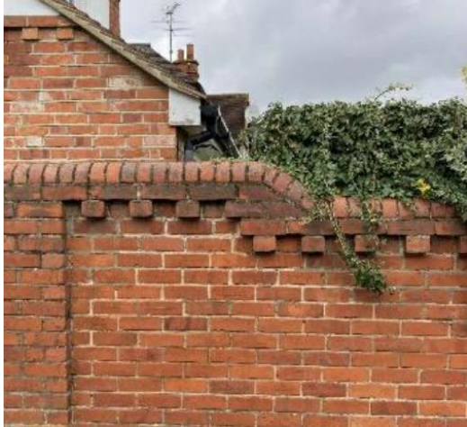
Photo of existing wall height difference
