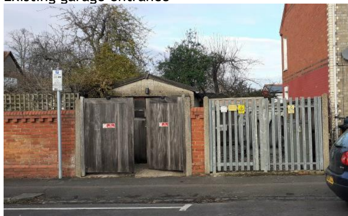
Existing garage entrance
