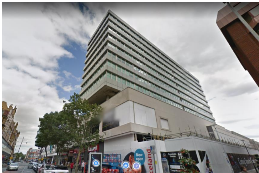
The application site
