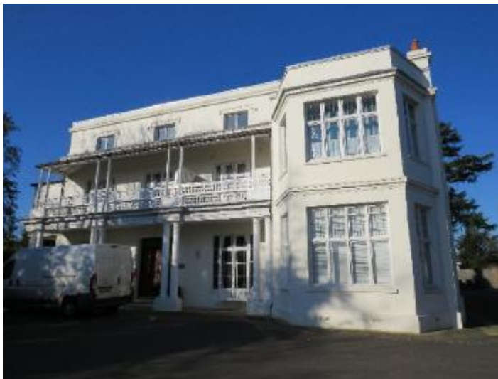
Photo 1 – View of the front elevation
