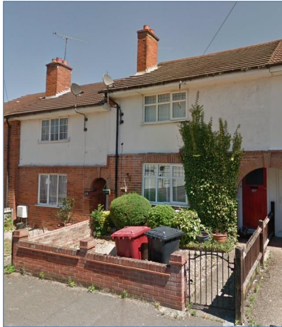
Fig. 1 - Google Street View image of 133 (left) and 135 (right) Wykeham Road. Image captured in June 2018.
