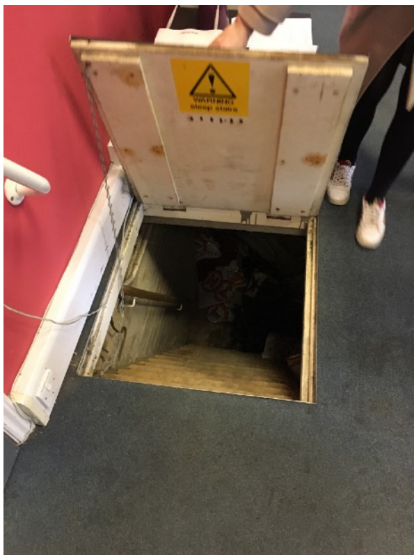
Existing hatch access to the basement from ground floor
