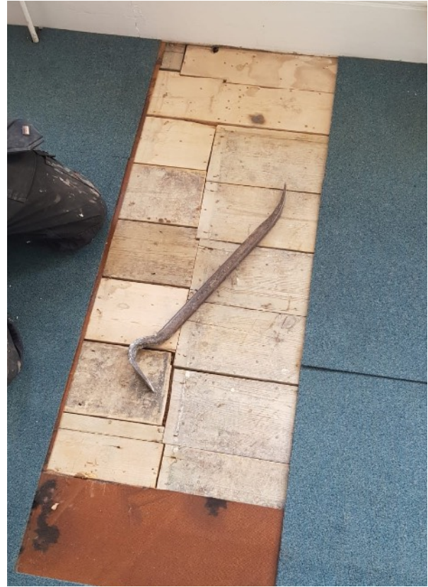
Photograph showing existing timber floor boards which will be made good and exposed as a feature. This small area shown was exposed for inspection purposes only.
