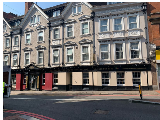
Fig 4: Royal Tandoori at ground floor with Ibis hotel directly above, opposite the site on Duke St.
