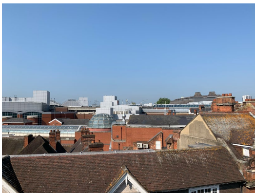
Fig 5: Roof of commercial properties at King's Walk and The Oracle, to the south-west of the site
