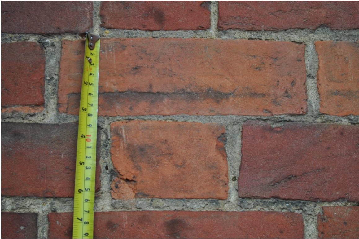
Fig 17 brick size and original lime mortar including visible grit.
