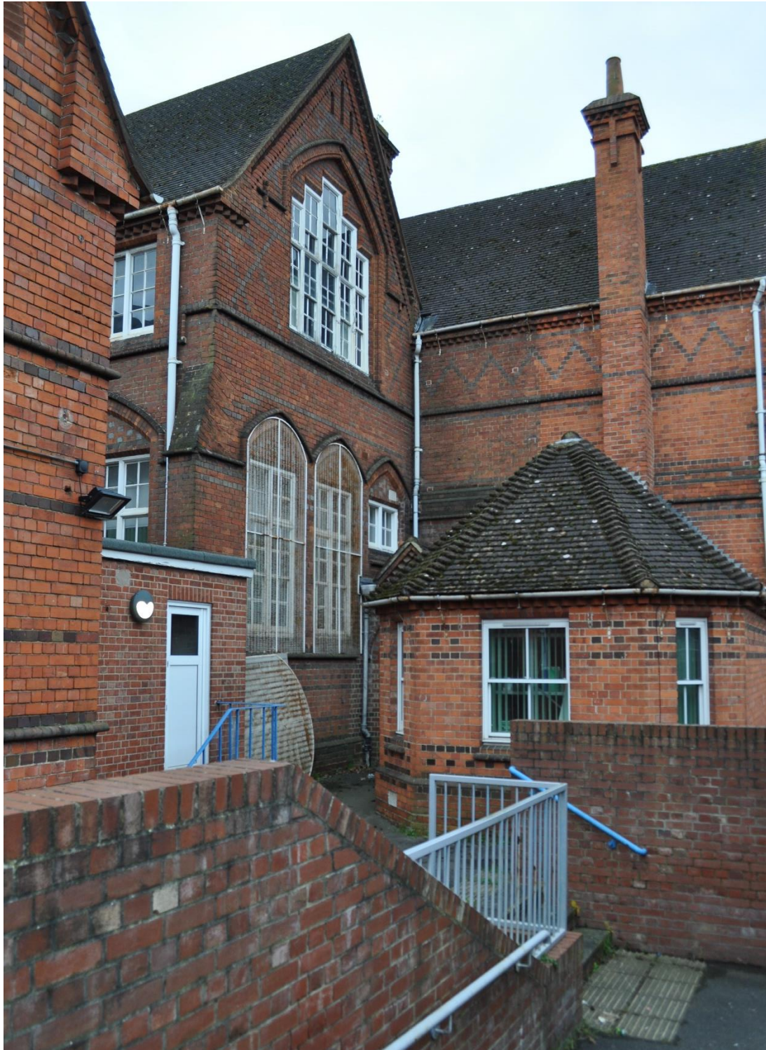
Fig 6 West elevation behind south wing Original timber windows in gable on the left.
