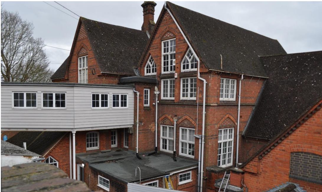
Fig 7 Two views of east elevation south and central wings with original timber windows
