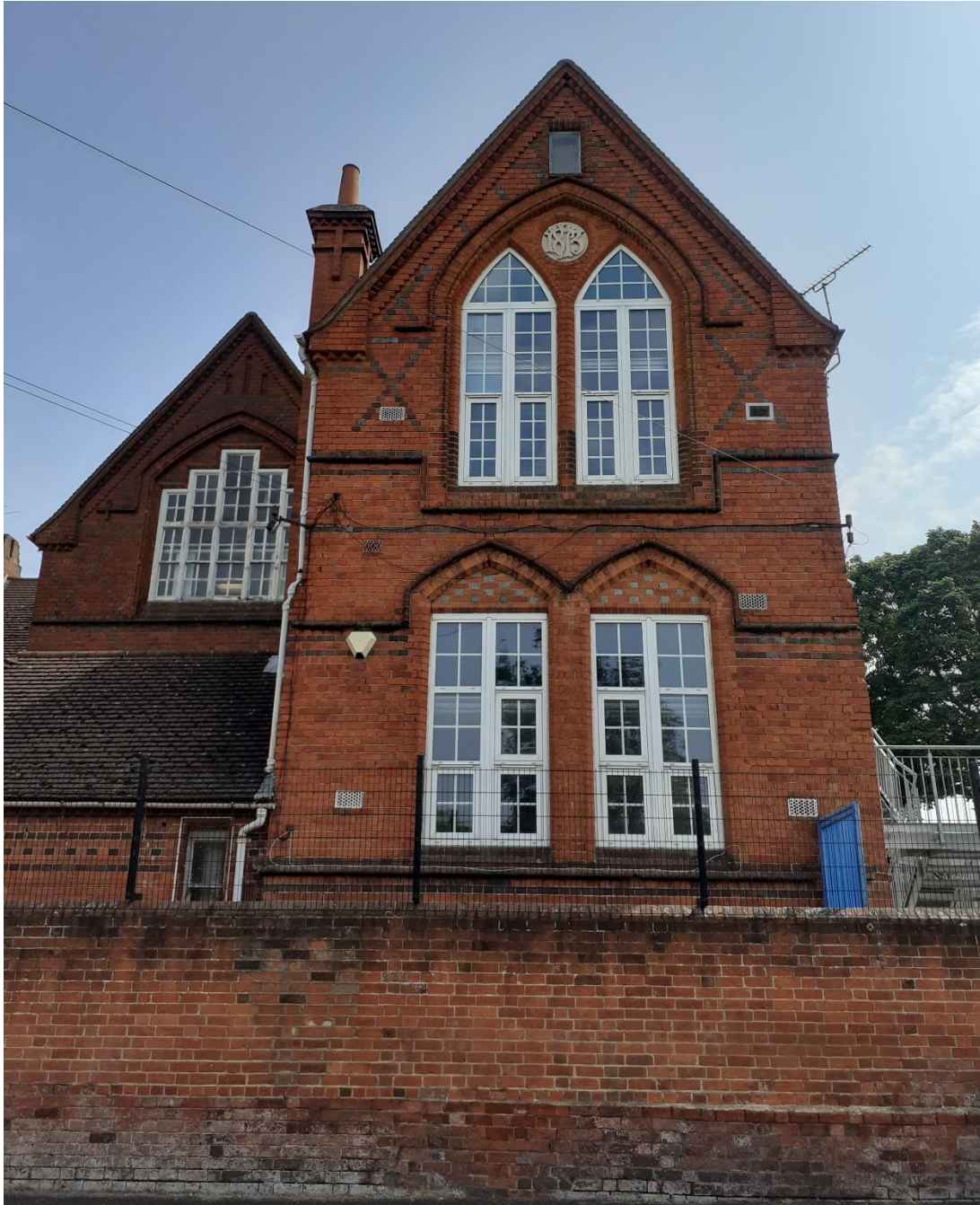
Fig 5 West side of south wing Modern replacement aluminium windows, original timber windows in gable on the left.
