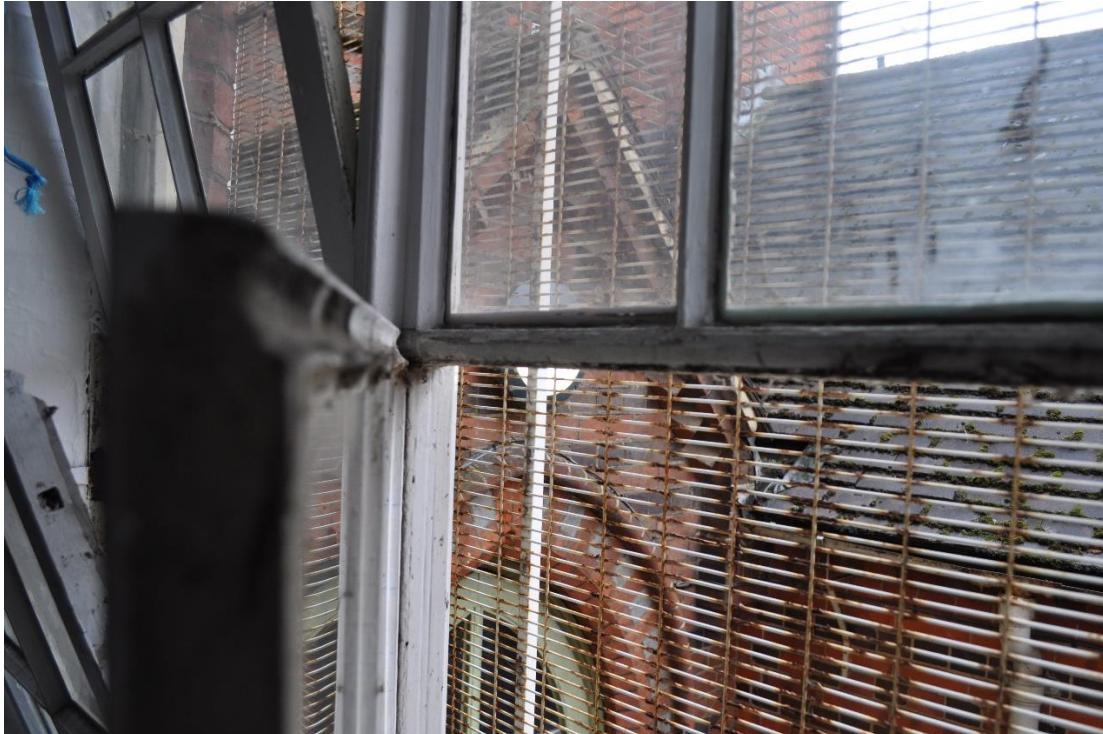
Fig 11 profiled meeting of head and cill normally where both bottom hung, here used in a side-hung format.
