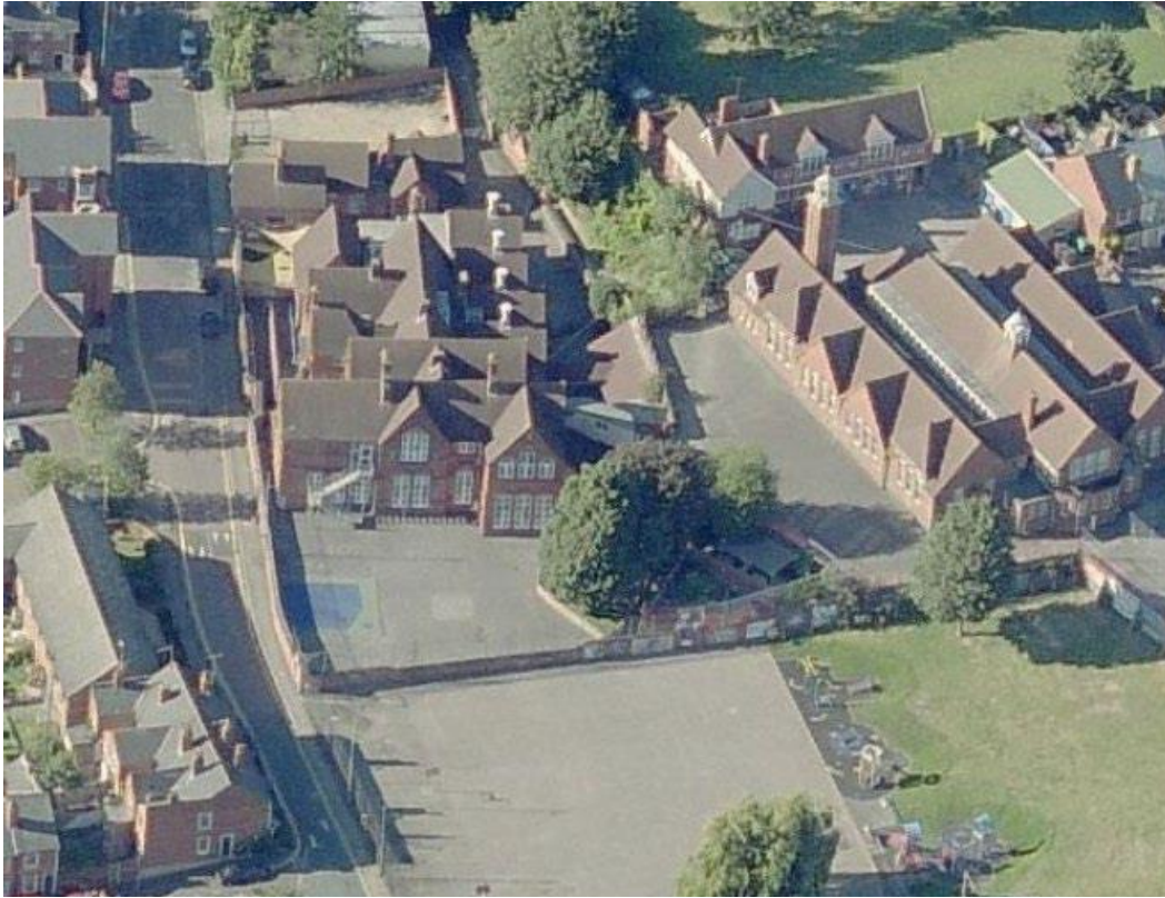
Fig 1: Aerial view of the Simmonds (Henry) Building from the South dating from the 1980s.
