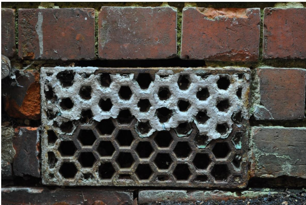
Fig 23 Cast iron air brick / ventilation grille at low level, high level ones similar design.
