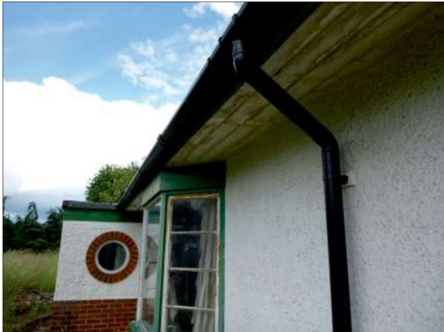
Photograph 2: Showing the well-sealed timber soffits/fascias.
