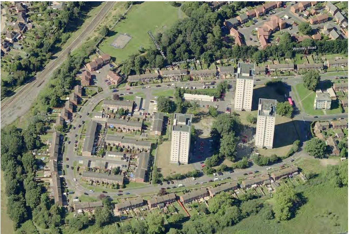
Figure 4 - Existing aerial photo from the South
