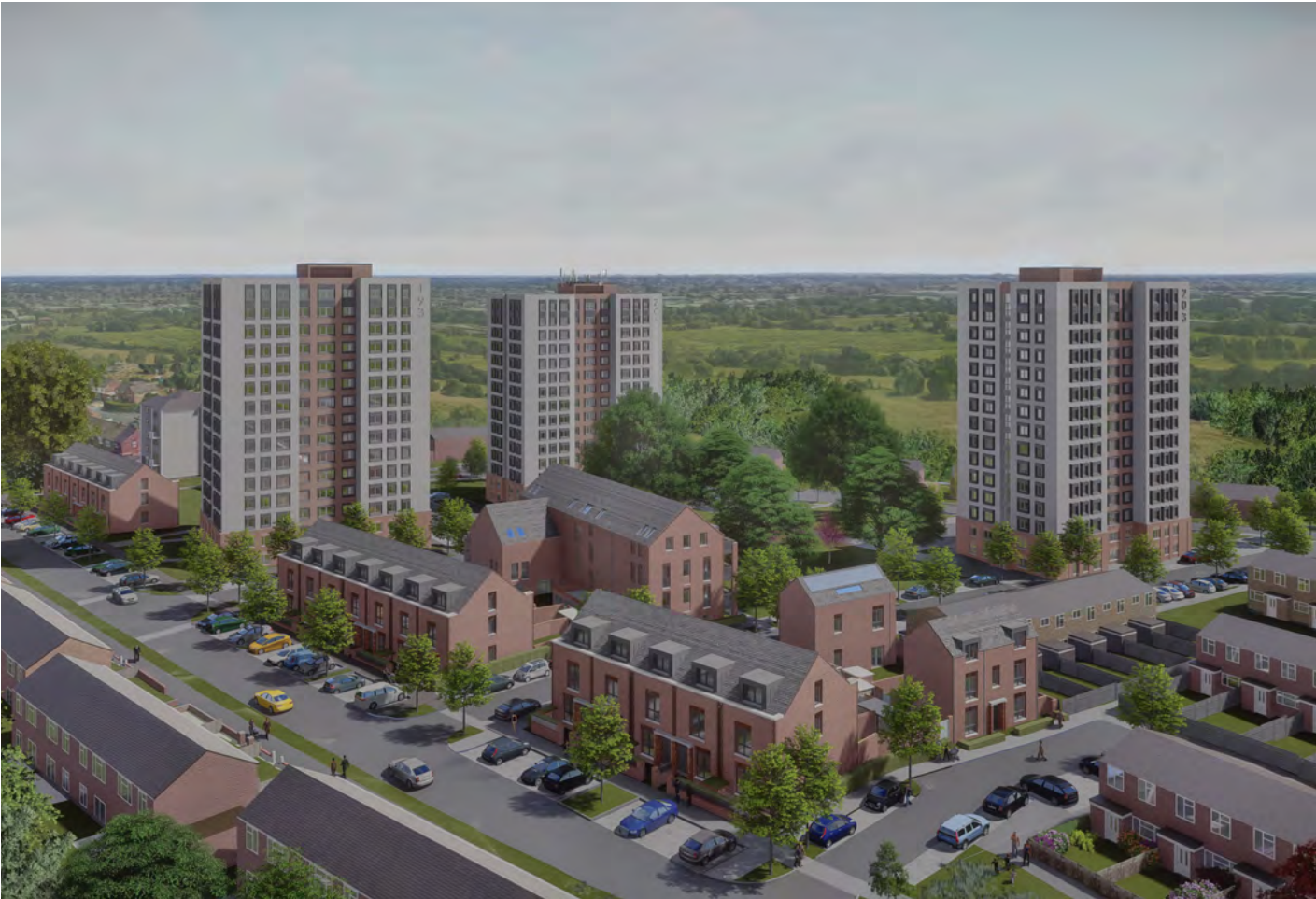
Figure 1 -Aerial view of the site, which includes Phase 1
