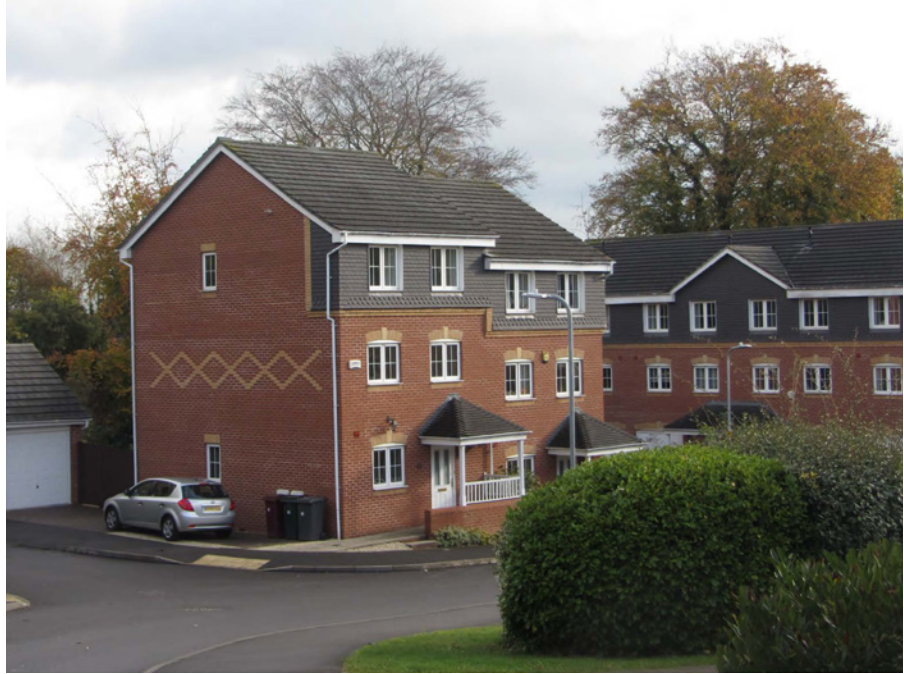
2. The image above shows a more recent (2002) residential dwelling located on Ruskin. The building is 3 storey with a change of material at the upper level fronting onto the main road.
