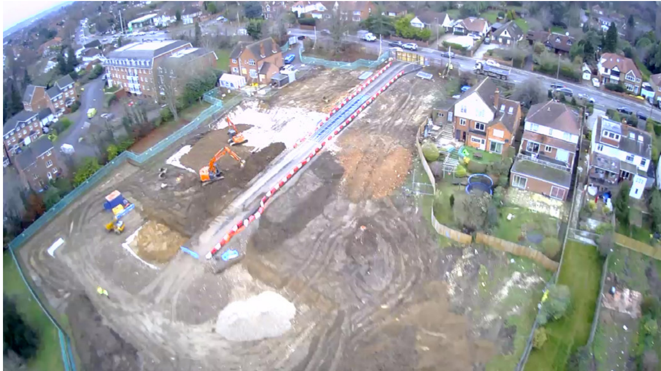
Aerial Image 2: Recent photo showing adjacent scheme under construction.
