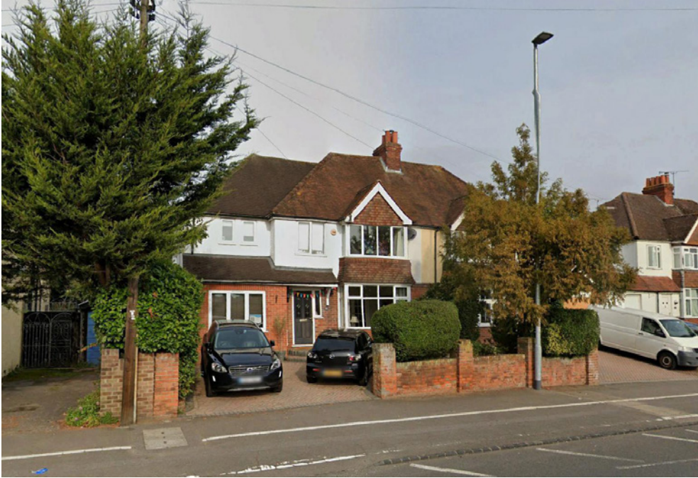
1. The image above is a typical 1930s house with a more recent two storey side extension which is a common characteristic of properties along the northern side of Henley Road. This house is constructed with a red brick base and a white render upper floor which may have been applied at a later date in-line with surrounding properties.
