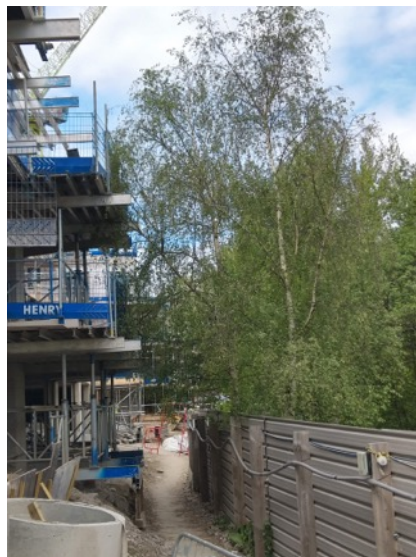
Photo 3: showing the minor contact between scaffolding and offsite silver birch trees.
