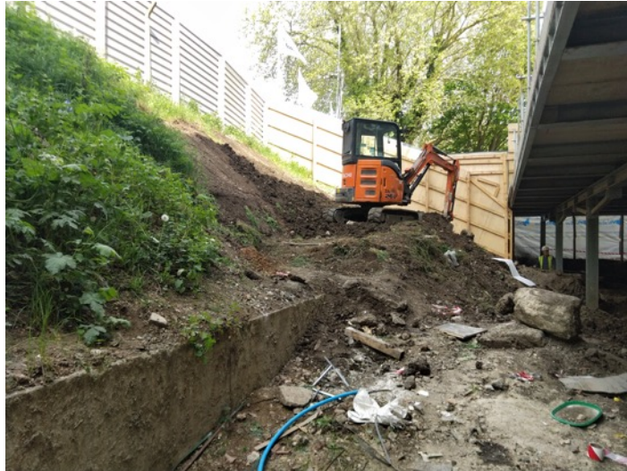
Photo 5: showing the regrading work required to the embankment down to the edge of the parking bays and over the existing retaining wall. Note, this is not within the CEZ of T1.
