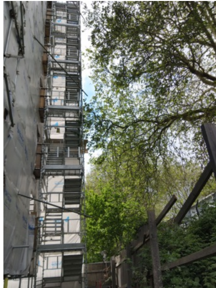
Photo 4: showing the minor contact between temporary access stairs and the crown of T1.
