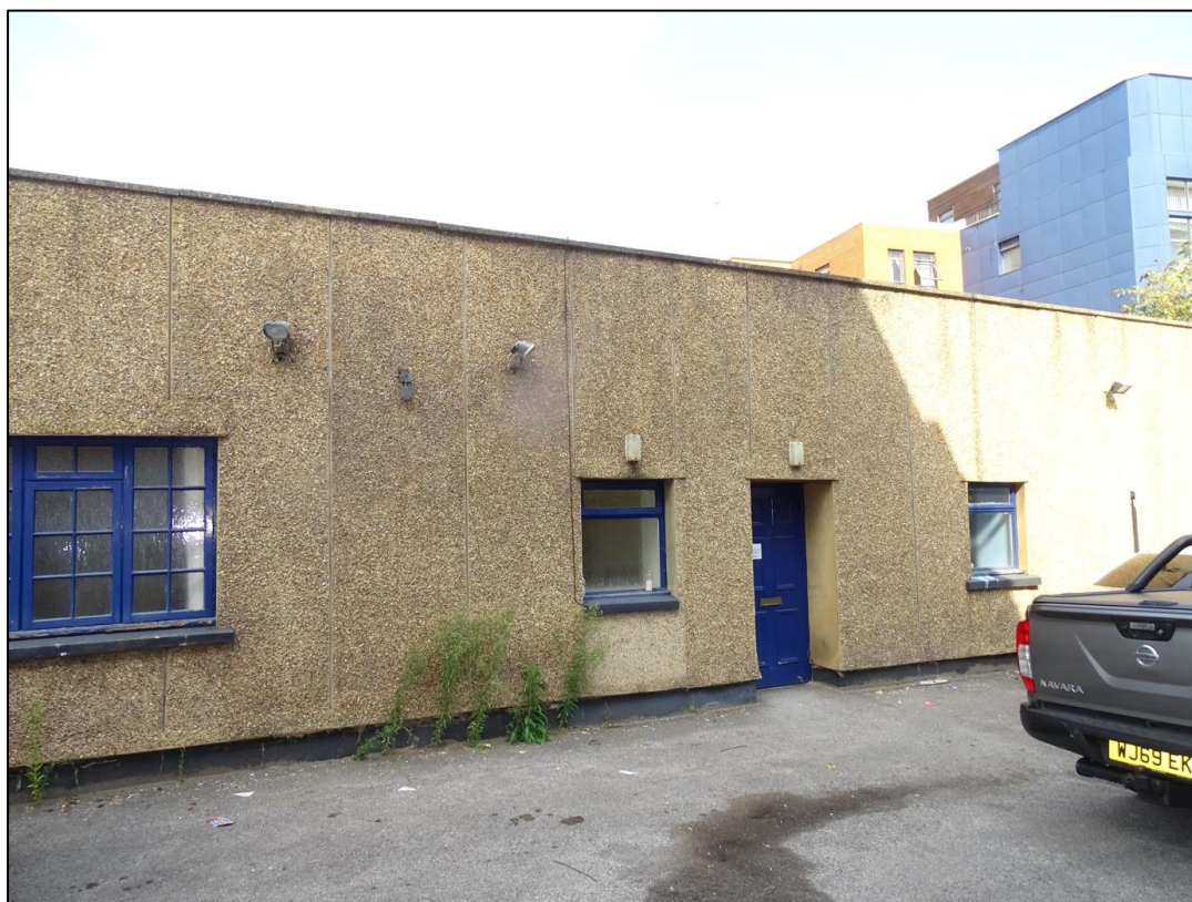
Photo 1: Southern elevation of building 1, taken facing northeast.
