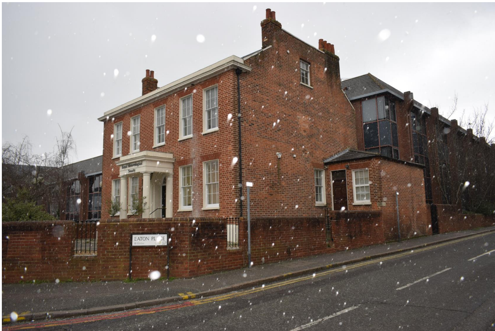
Plate 1: View of the front and side elevation of the building and extension
