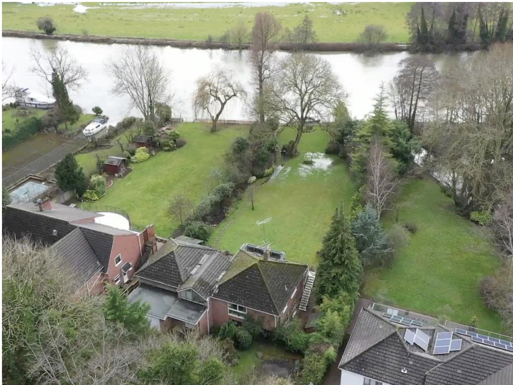
Aerial view of the property.
