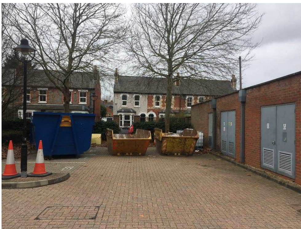
Plate 10 – North wester corner, Electrical hut and disposal material area.
