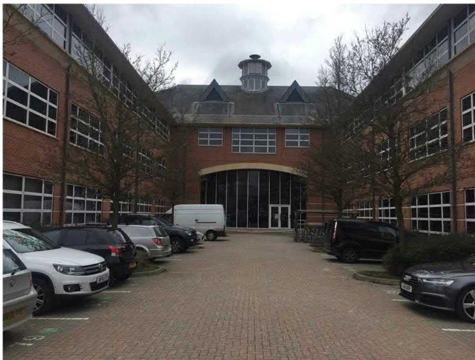
Plate 9 – North facing entrance of GBM building.
