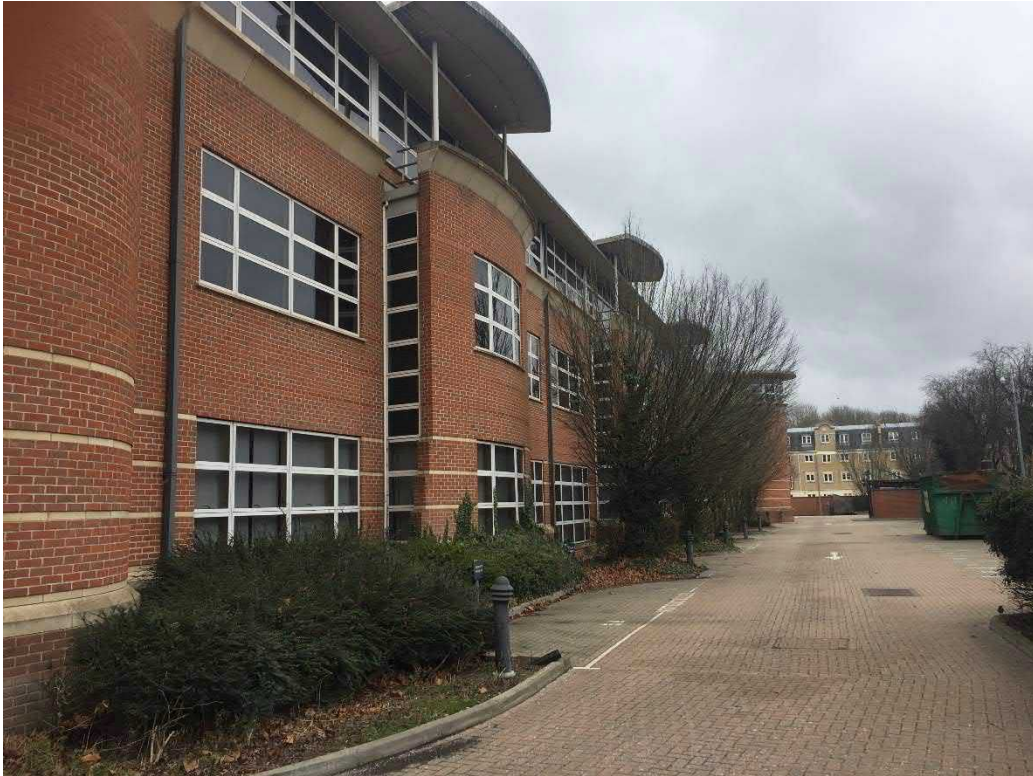
Plate 5 – East facing view of main GBM building.
