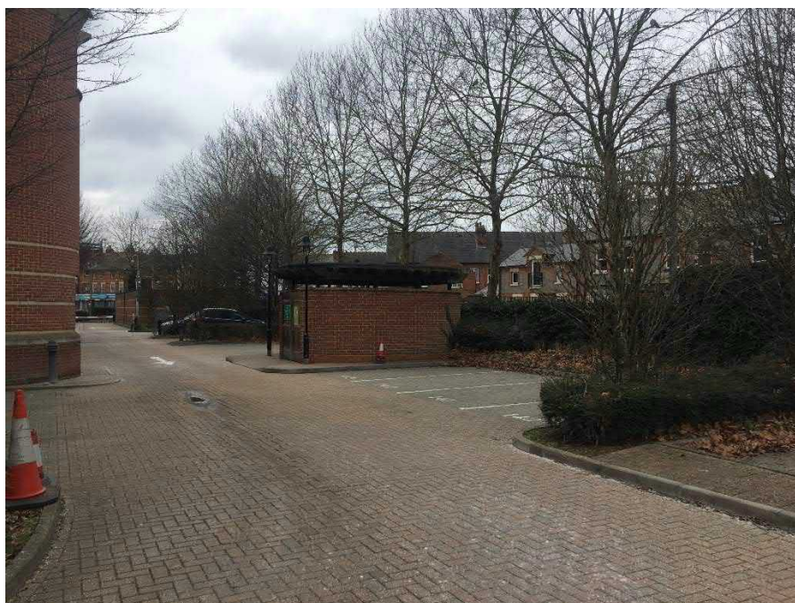
Plate 12 – West facing view of car park and landscaped area
