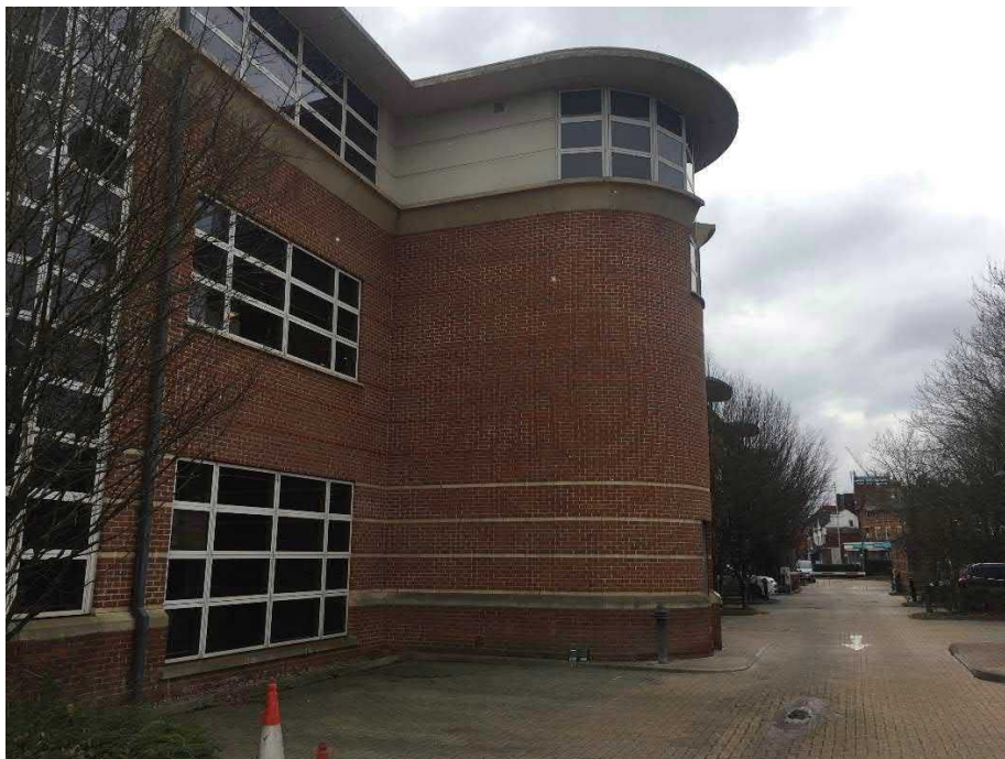
Plate 11 – West facing view of main GBM building.
