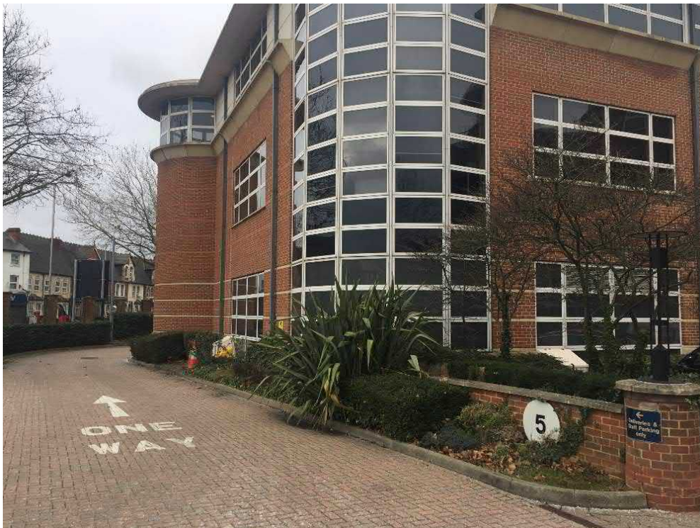
Plate 2 – South facing Car Park Entrance
