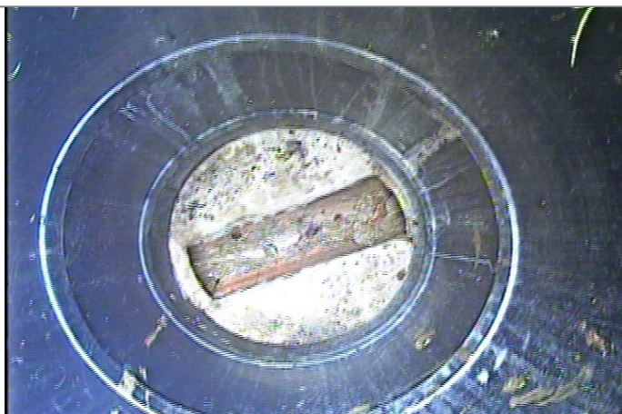
Manhole / Access Point: S5 TANK JETTING ACCESS POINT Internal
