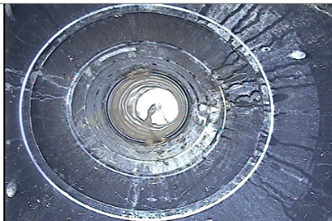
Manhole / Access Point: S2 Internal
