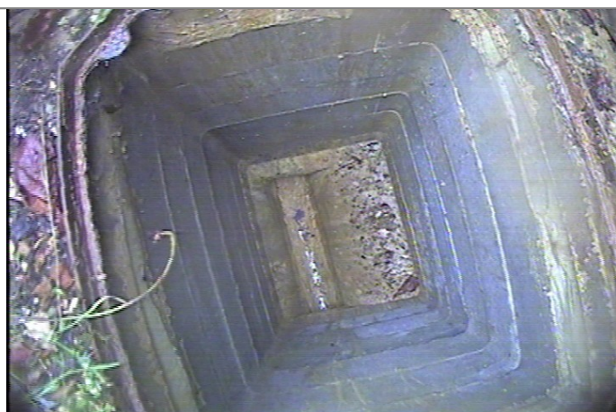
Manhole / Access Point: UPPER REDLANDS ROAD Internal
