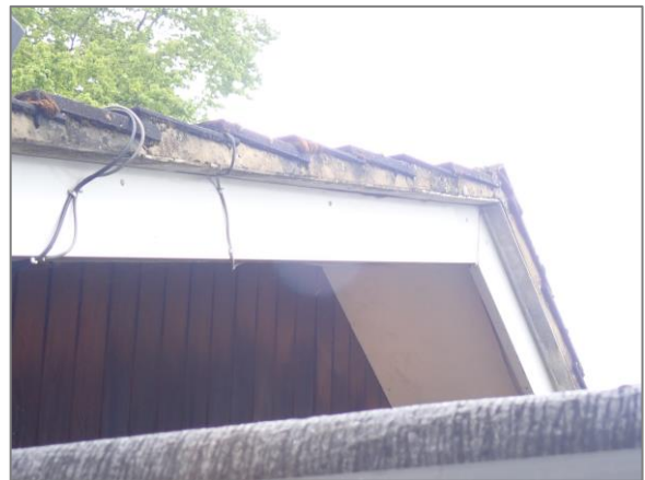
Photo 18 Verge mortar in good condition
