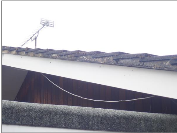
Photo 19 Verge mortar in good condition
