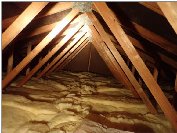
Photo 3 General conditions in main loft
