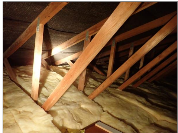
Photo 4 General conditions in main loft
