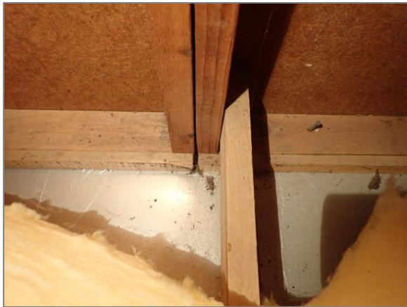
Photo 9 Floor beneath gable apex
