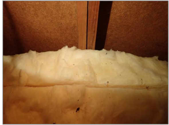
Photo 8 Top of insulation below gable end
