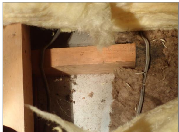
Photo 6 Spot checks beneath insulation
