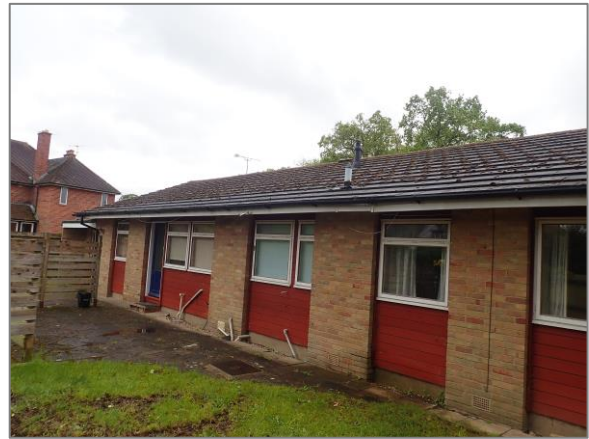
Photo 2 Rear of house
