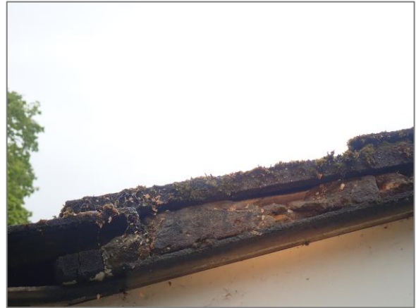
Photo 20 Gap to verge mortar
