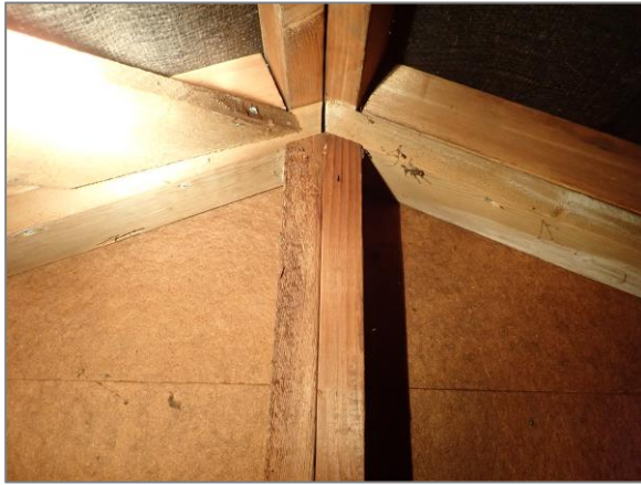
Photo 7 Gable end apex
