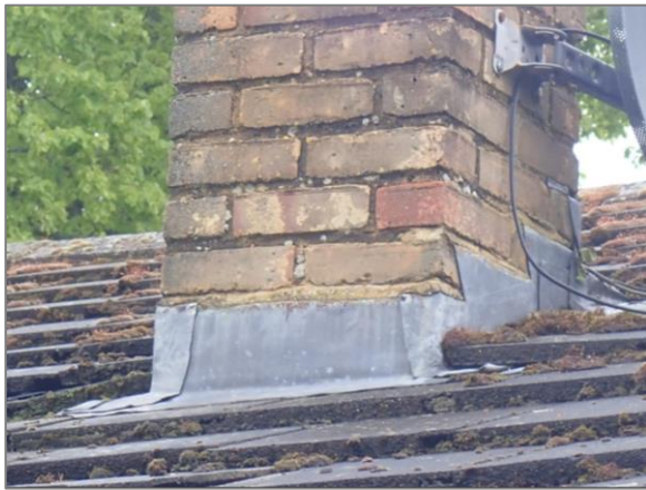
Photo 15 Chimney flashing
