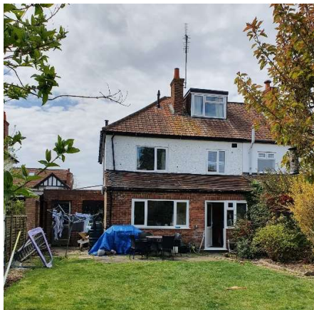
Rear elevation, showing the existing extension to be replaced.
