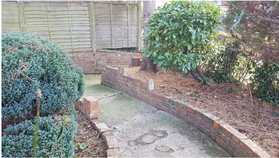
Photo 2 – Brick edging and concrete path to be removed at front of property.
