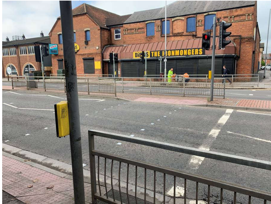
Photograph 2.3: Signalised Crossing at Caversham Road
