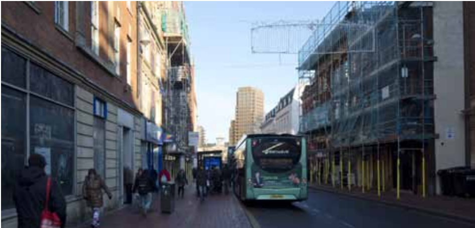
Residential Building on Plot D
