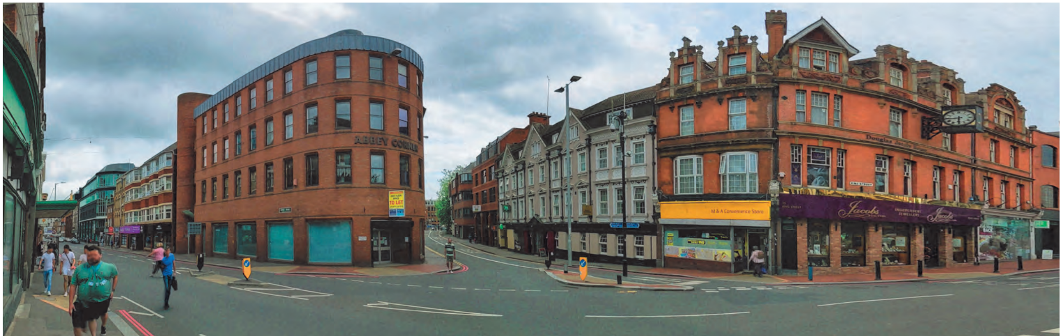
Figure 1: Kings' Road Streetscene showing the site and street context.
