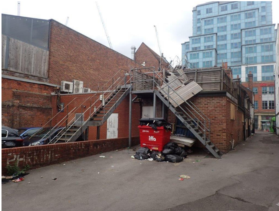
Photograph 7: Rear of the buildings at Friar Street Reading.
