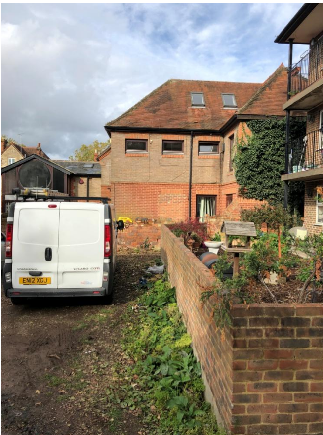
View from car park towards rear of No. 4 and existing garden
