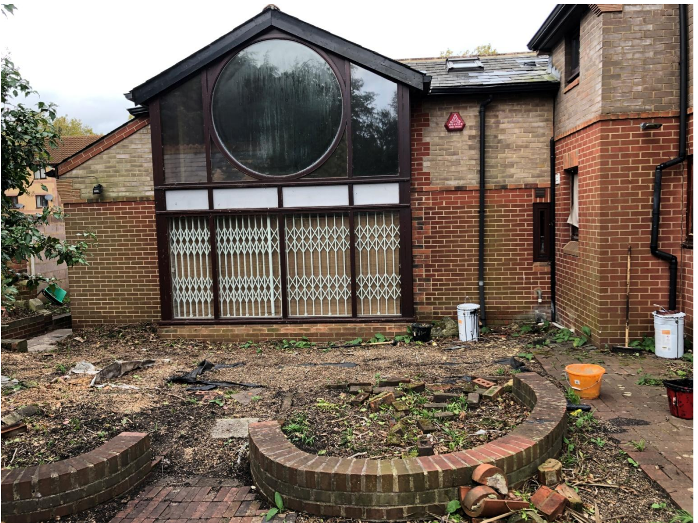
Existing rear garden at 2-4 Alexandra road
