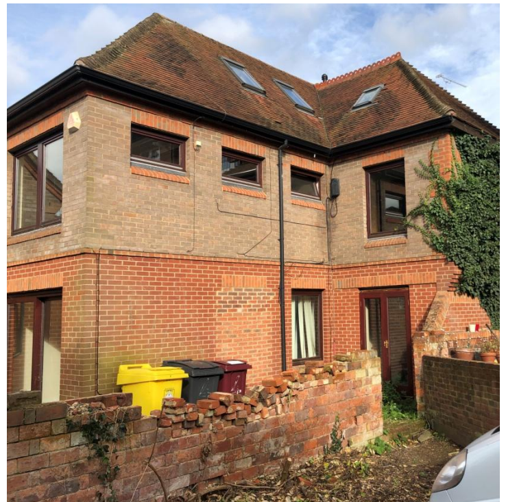
Side and rear elevation of No. 4 showing low boundary wall within the conservation area
