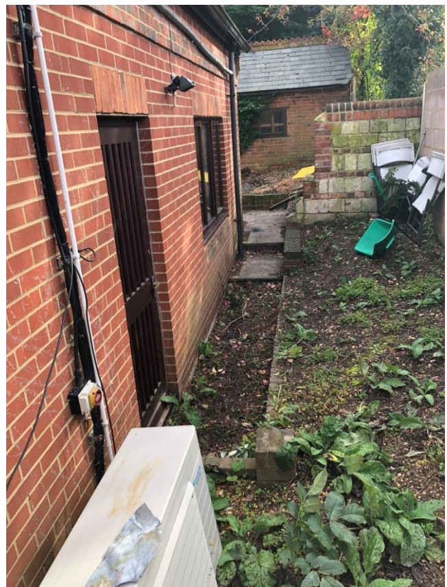
View from rear exit door at No. 2 towards existing rear garden
