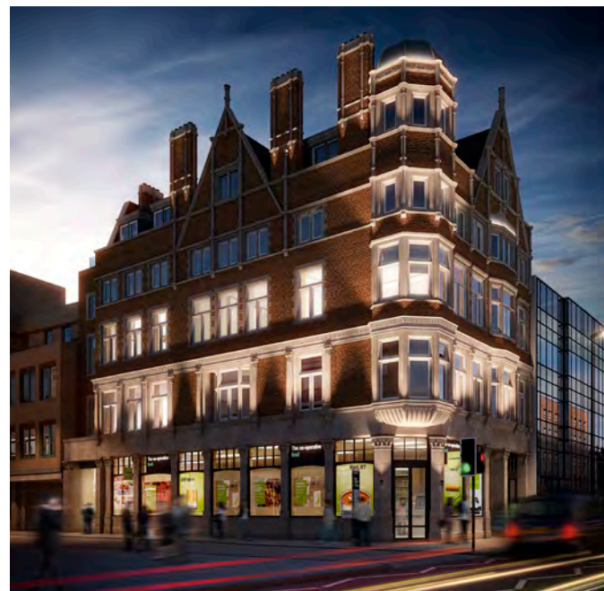
Dover House, Waterloo, London
