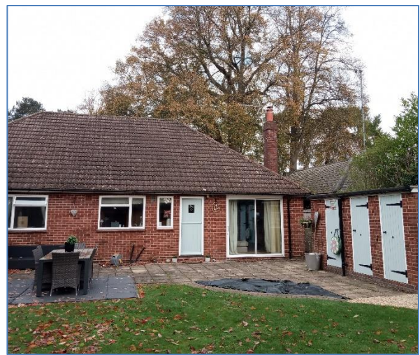
Fig 2. Rear of 18 Richmond Road. Site photo taken by case officer on 03/11/2021
