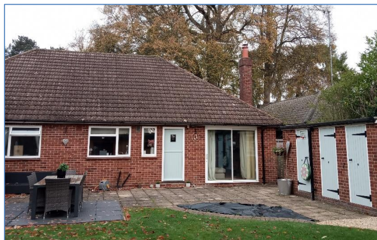
Fig 3. Rear of 18 Richmond Road, garden storage building to be demolished pictured to the right of the photo. Site photo taken on 03/11/2021 by case officer.
