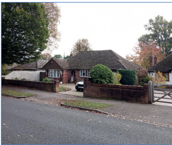
Fig 1. Front of 18 Richmond Road. Site photo taken by case officer on 03/11/2021
