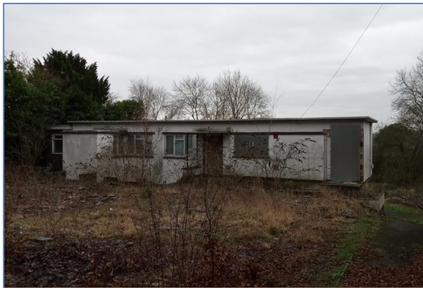
Fig 1. Existing front elevation. Site photo taken on 06/01/2022.
