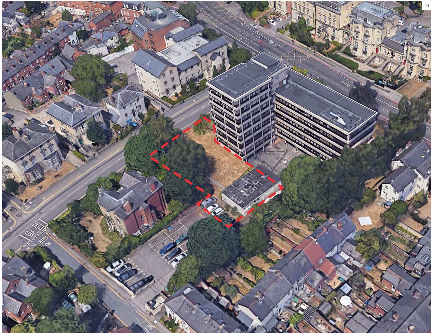
01 3D view of the site showing the recently demolished dental surgery (looking north-west)
