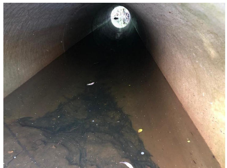
Figure 2: Culvert view Western Boundary
