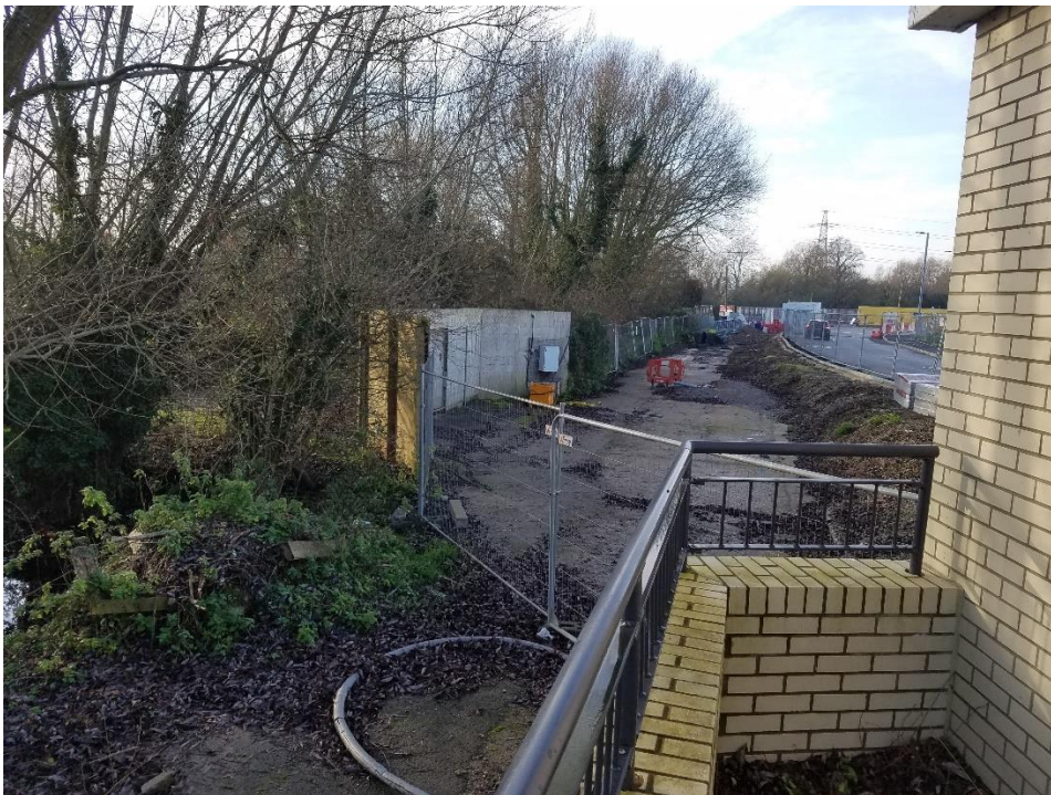
View across culvert, looking west, showing difference in level to the newly built road
