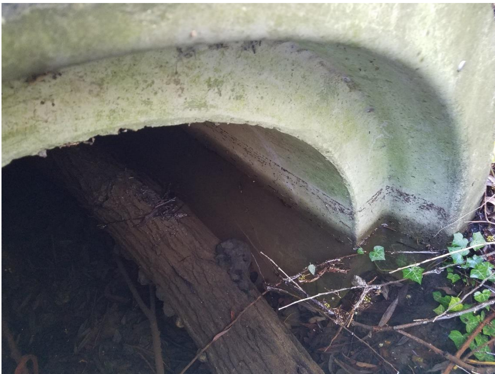
Western end of culvert
