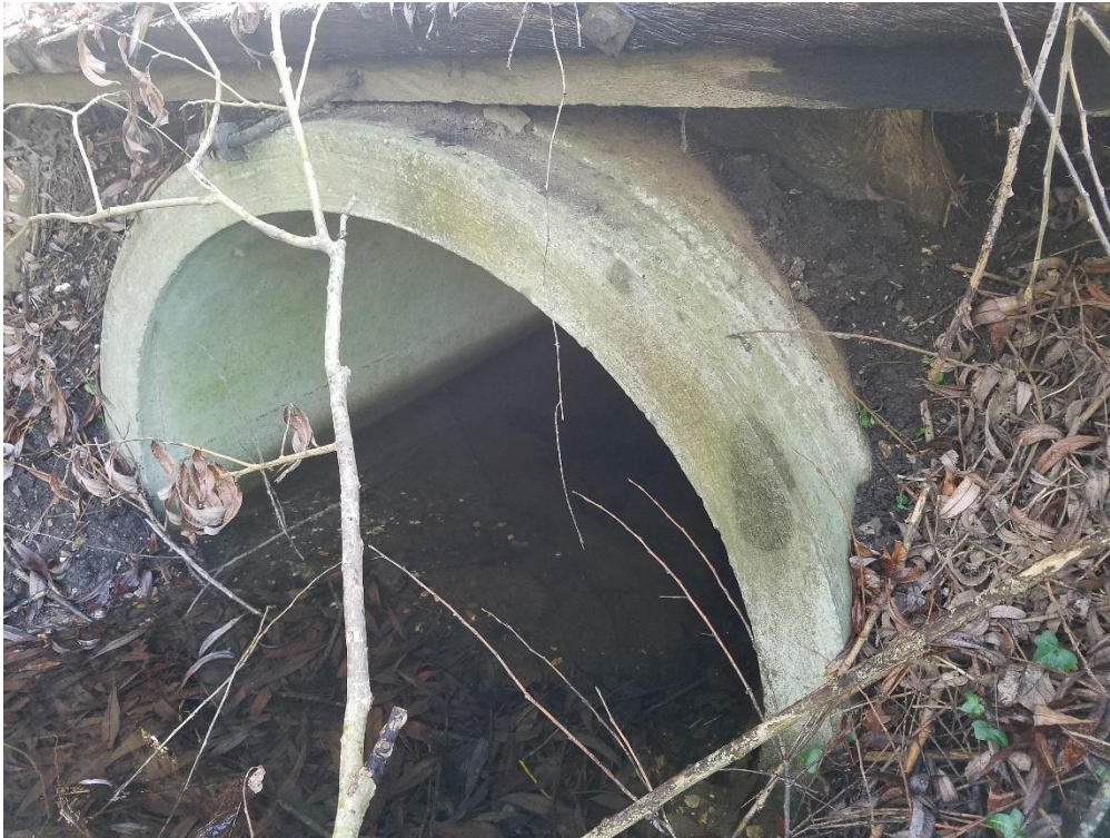
Eastern end of culvert
