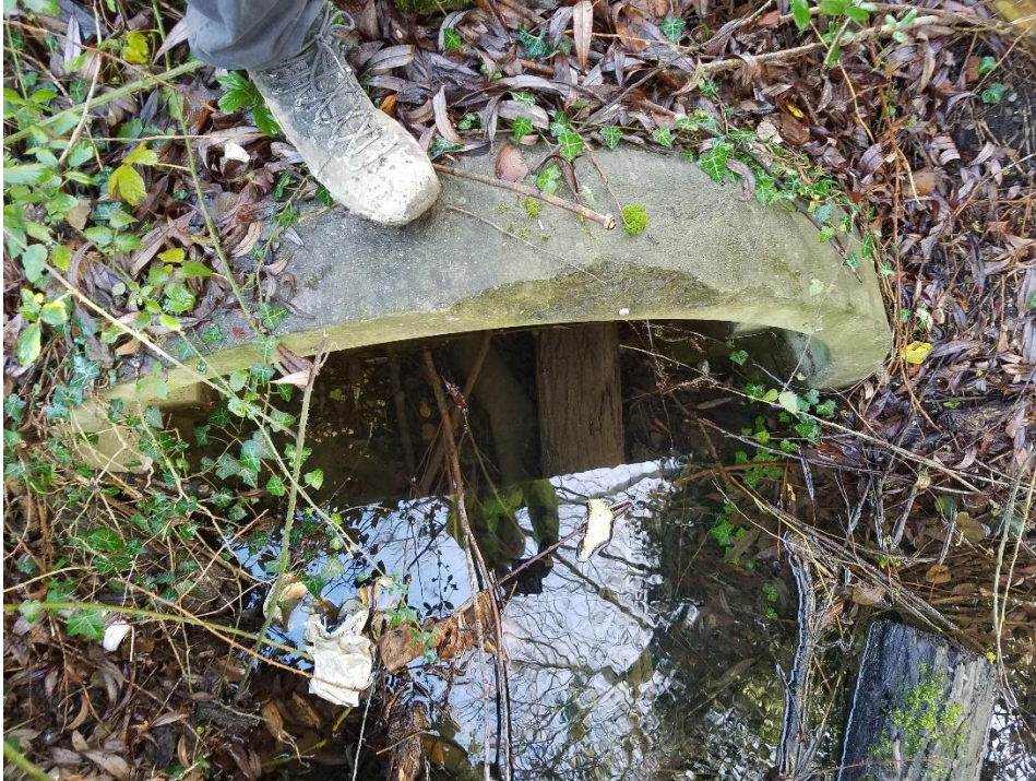
Western end of culvert
