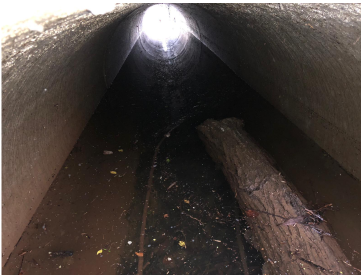
Figure 1: Culvert view Eastern Boundary
