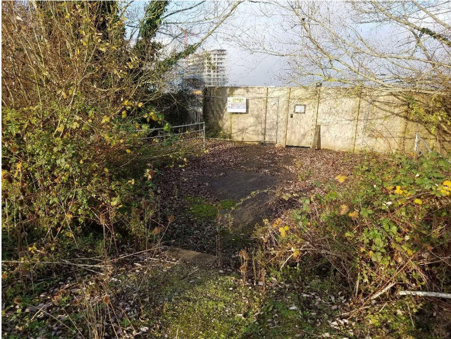
View across existing crossing, towards north-west
