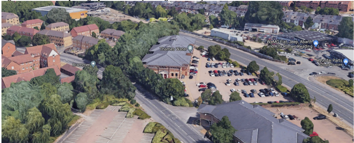
Figure 2.6: 3D aerial photograph of the site (looking northeast)
