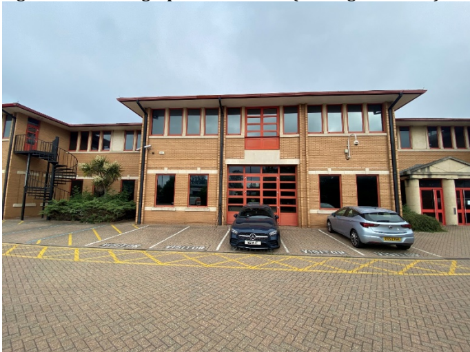
Figure 2.13: Photograph from outside (looking northeast)
