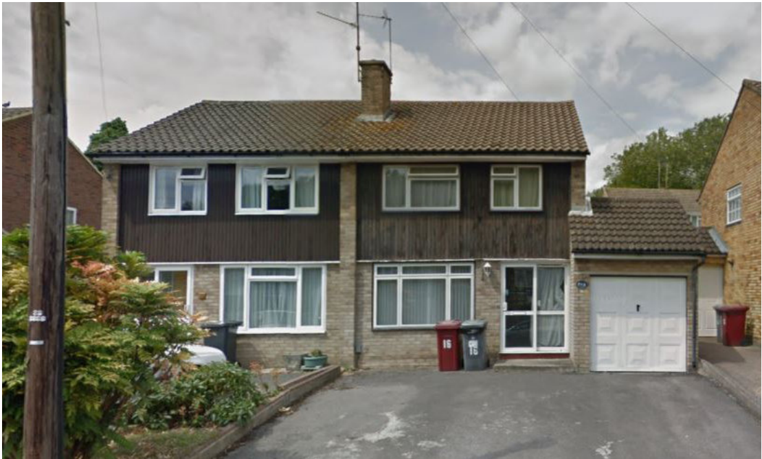
Timber cladding finish at No.16, No.18 Trelleck Road
