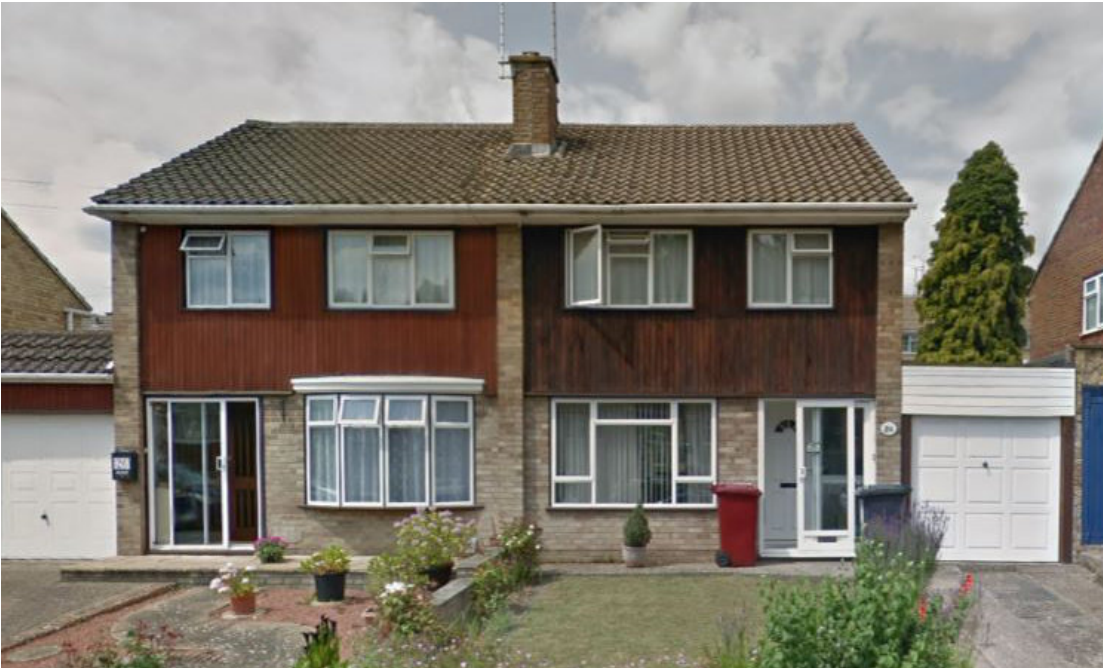
Timber cladding finish at No.24, No.26 Trelleck Road
